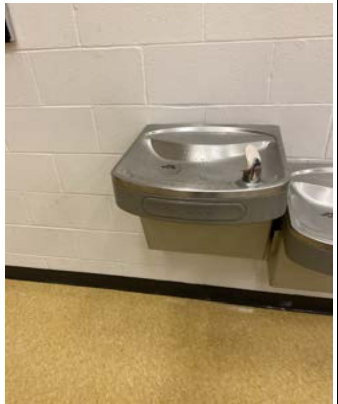
1/9/2024 - 3000-50 - Bell Prairie Elementary - Cafeteria-Left
