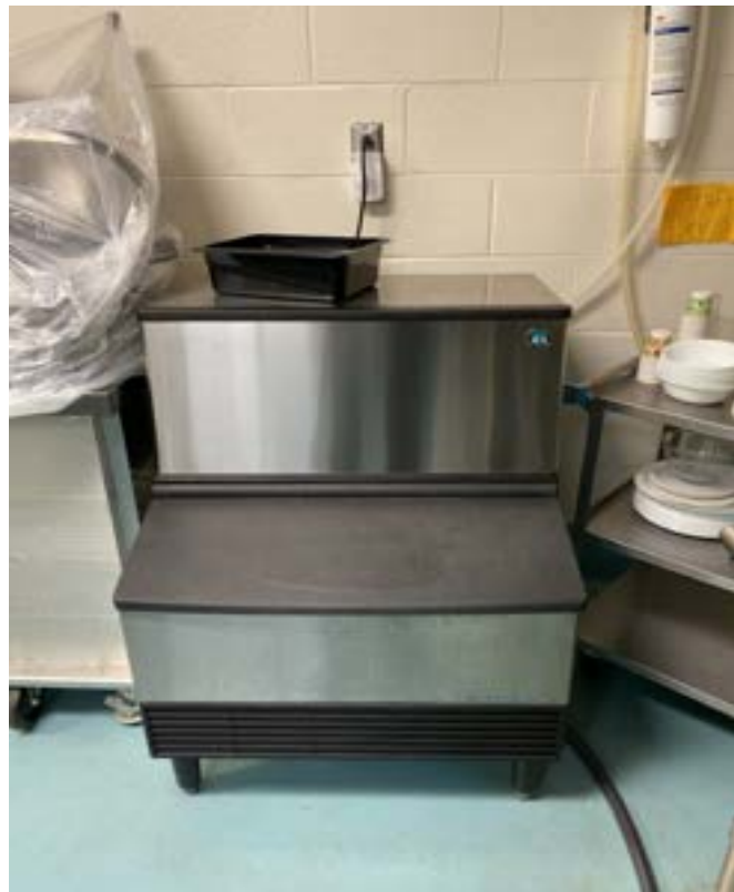
1/9/2024 - 3000-61 - Bell Prairie Elementary - Kitchen
