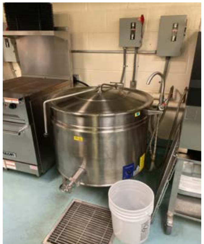
1/9/2024 - 3000-56 - Bell Prairie Elementary - Kitchen
