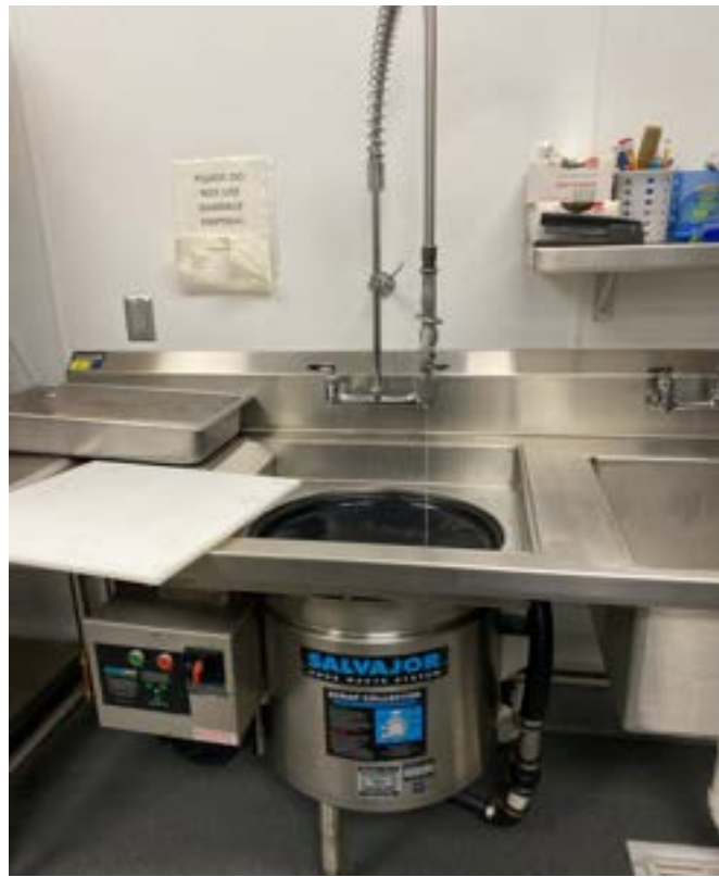
1/12/2024 - 5100-33 - Davidson Elementary - Kitchen-North Wall-Left
