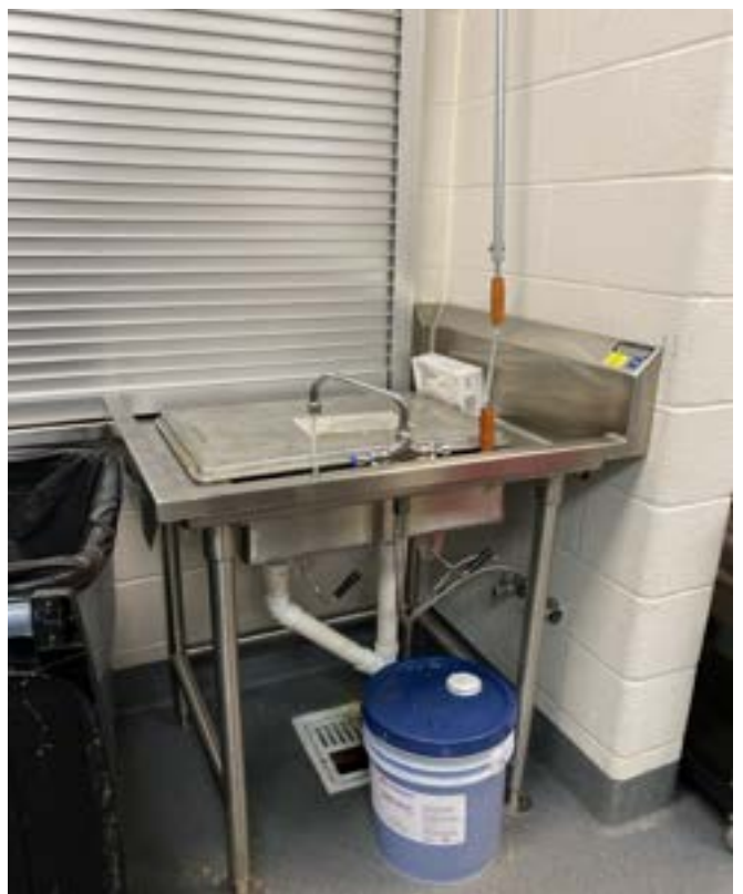
1/12/2024 - 5100-36 - Davidson Elementary - Kitchen-South Wall
