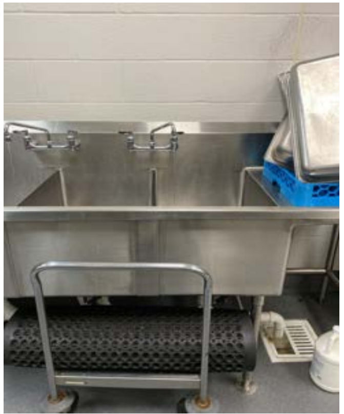
1/12/2024 - 5100-34 - Davidson Elementary - Kitchen-Three Bay Sink-Right
