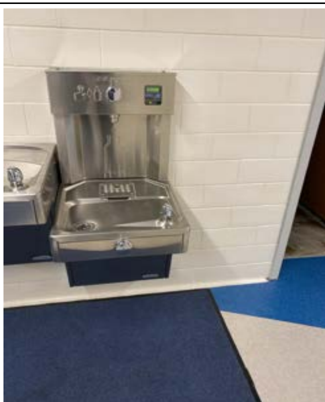
12/28/2023 - 4100-34 - Briarcliff Elementary - Outside Office-Right
