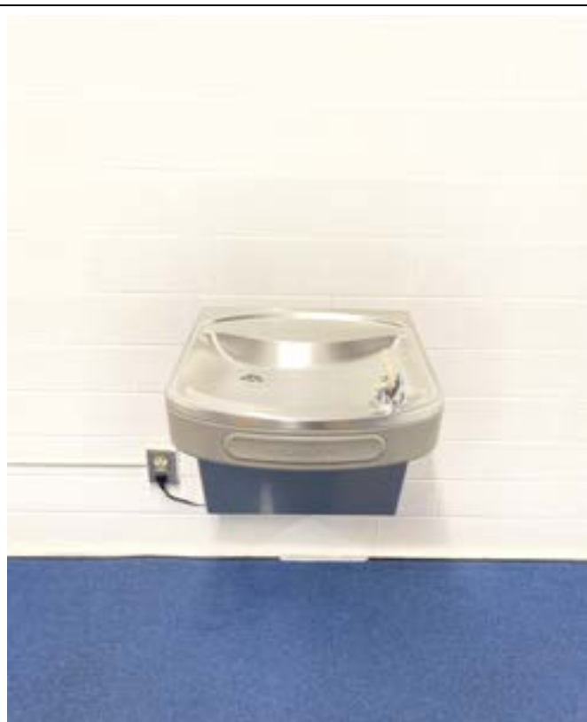
12/28/2023 - 4100-47 - Briarcliff Elementary - Outside Room 8
