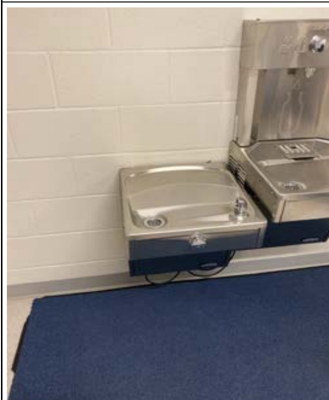
12/28/2023 - 4100-35 - Briarcliff Elementary - Restrooms by Room 5-Left
