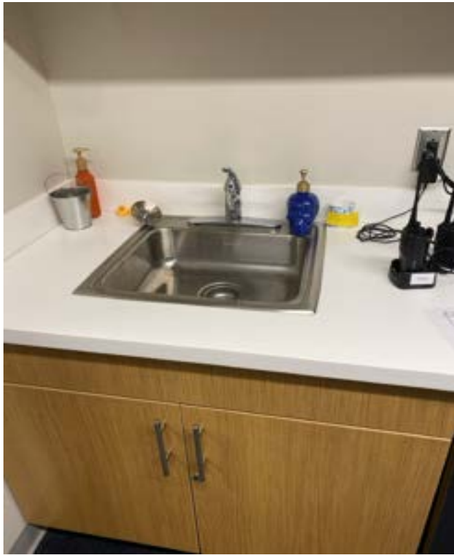
12/28/2023 - 4100-1 - Briarcliff Elementary - Office Sink
