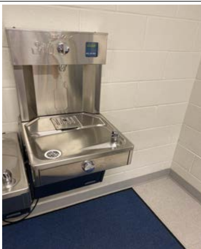
12/28/2023 - 4100-36 - Briarcliff Elementary - Restrooms by Room 5-Right
