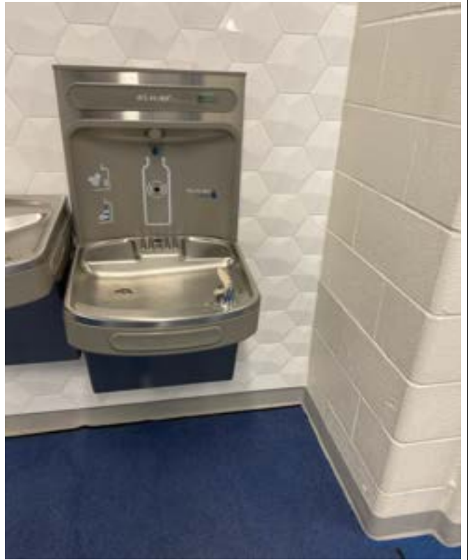
12/28/2023 - 4100-26 - Briarcliff Elementary - Outside Gym-Right
