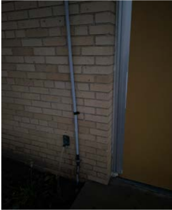
12/28/2023 - 4100-53 - Briarcliff Elementary - Outside Door 3
