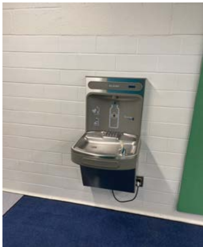
12/28/2023 - 4100-7 - Briarcliff Elementary - Outside Room 21
