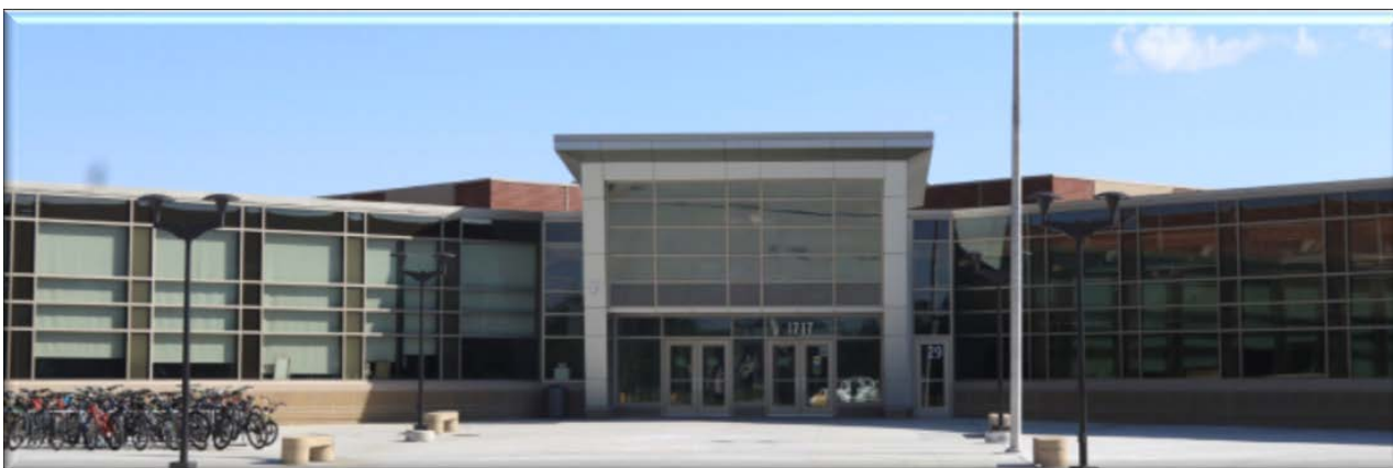
Discovery Middle School Entrance After
