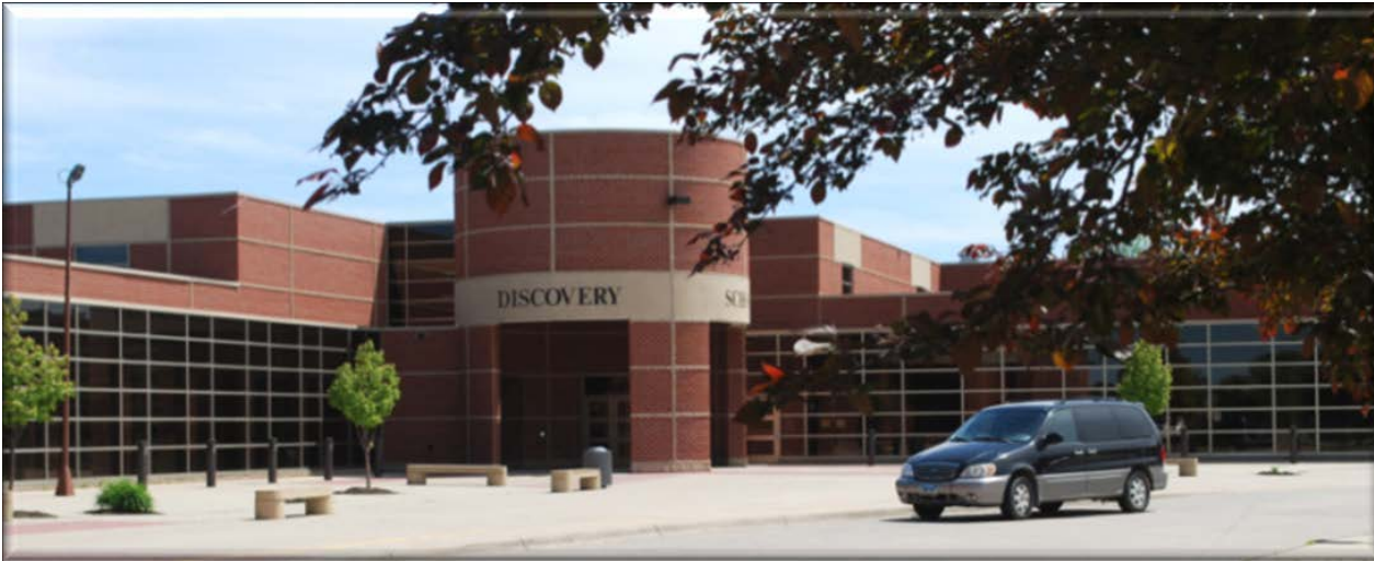
Discovery Middle School Entrance Before
