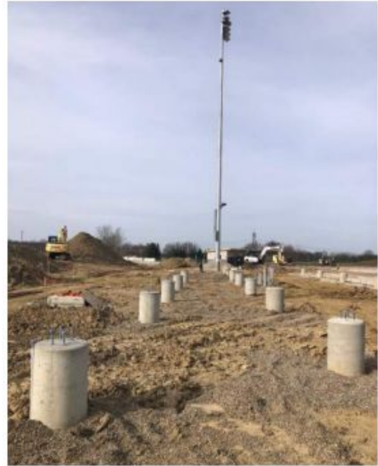
03.12.24 - Foundation Piers for Home Grandstand
