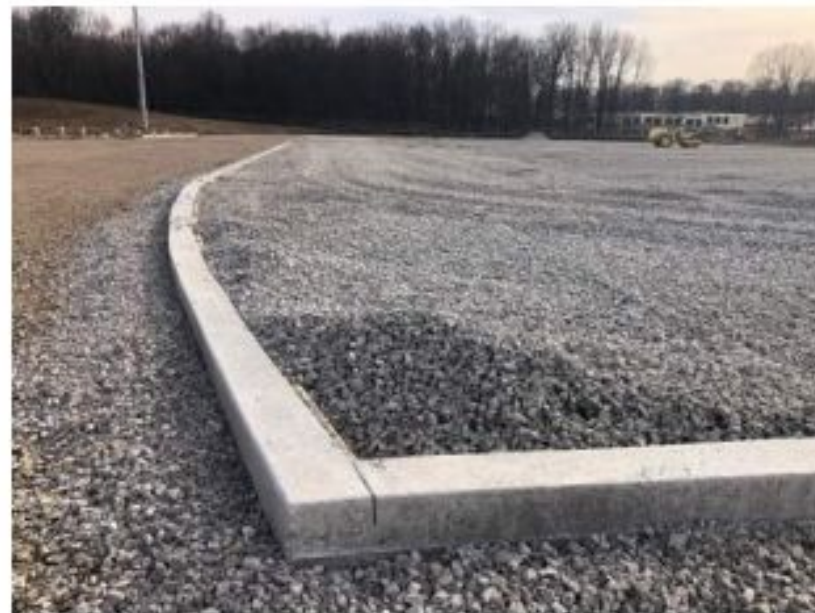
03.12.24 - Concrete Curb at Synthetic Turf Field
