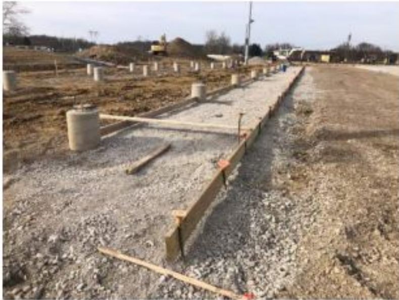
03.12.24 - Form Concrete Walk at Home Grandstand
