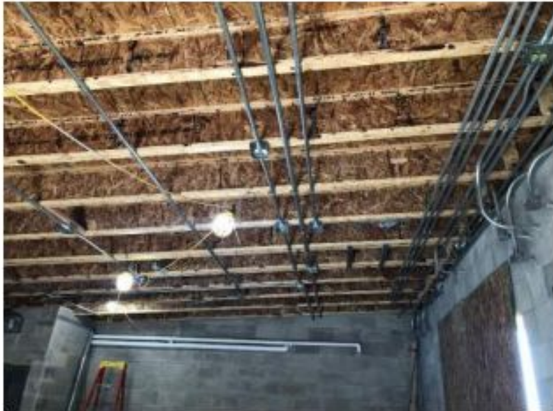
03.12.24 - Electrical Overhead Rough-in at Concession Stand
