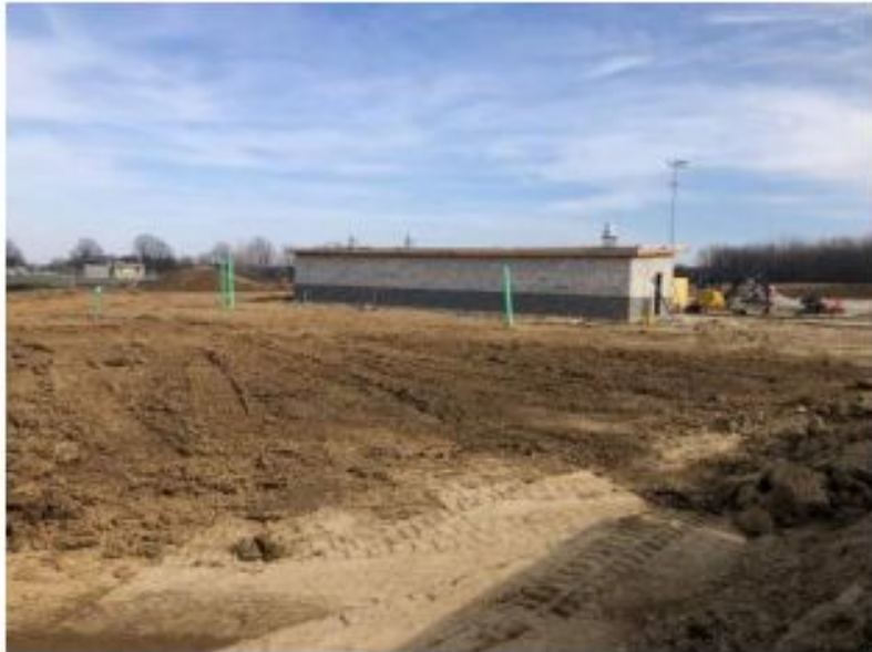
03.12.24 - Temporary Sediment Basin Backfilled
