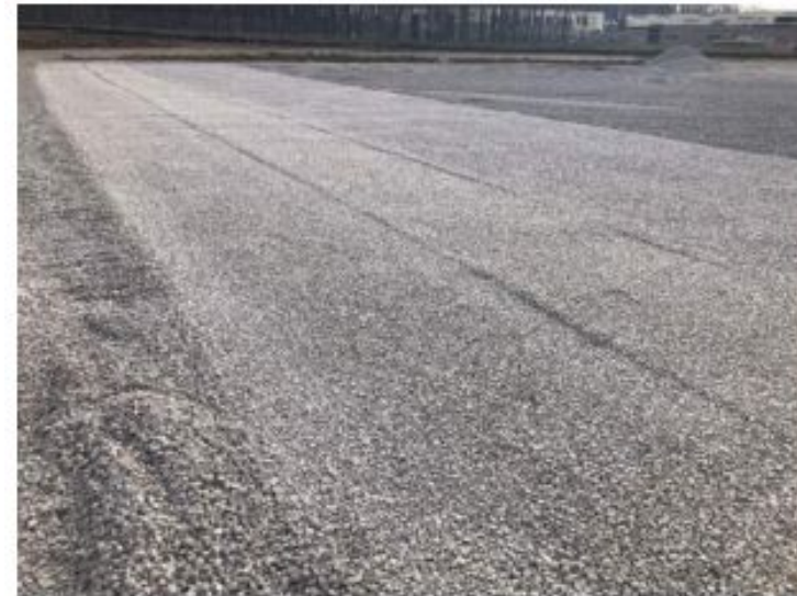
03.12.24 - Fine Grade Stone base at Synthetic Turf Field
