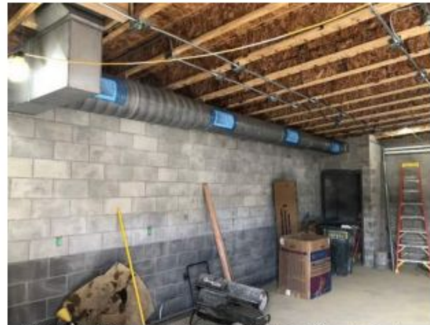
03.12.24 - Overhead HVAC and Electrical Rough-in at Concession Stand
