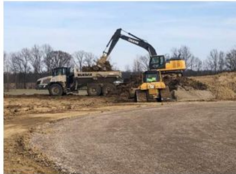
03.12.24 - Removing the remaining stockpile soil on site
