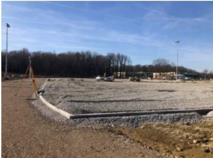
03.12.24 - Concrete Curb and Fine Grading at Synthetic Turf Field
