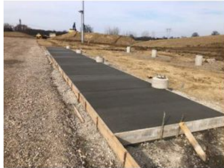
03.12.24 - Place Concrete Walk at Visitor Grandstand
