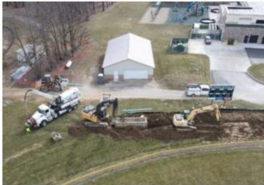
02.12.24 - Water Line for Concession Stand
