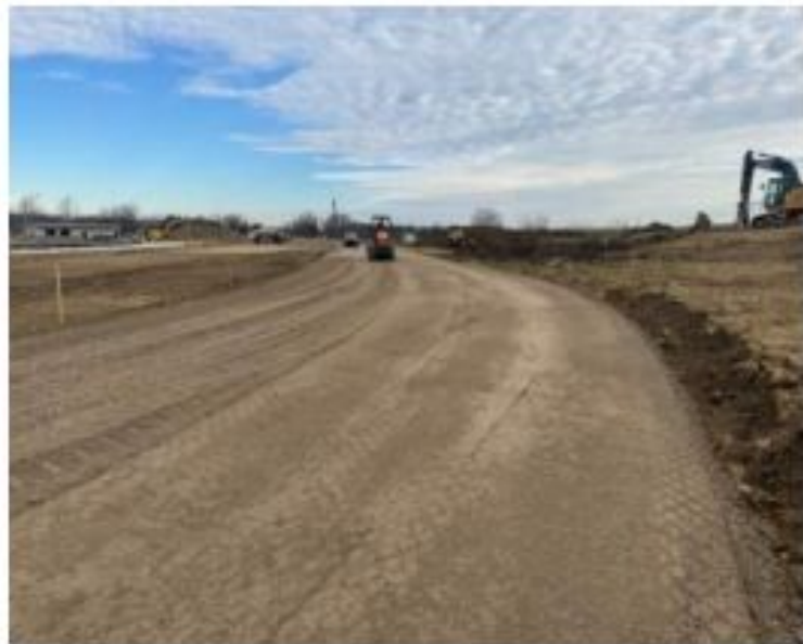
02.08.24 - Place and Compact 6" of stone Base at Track
