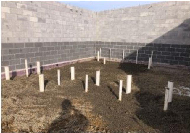
01.05.24 - Masonry Bearing Walls & Underground Plumbing at Concession Stand
