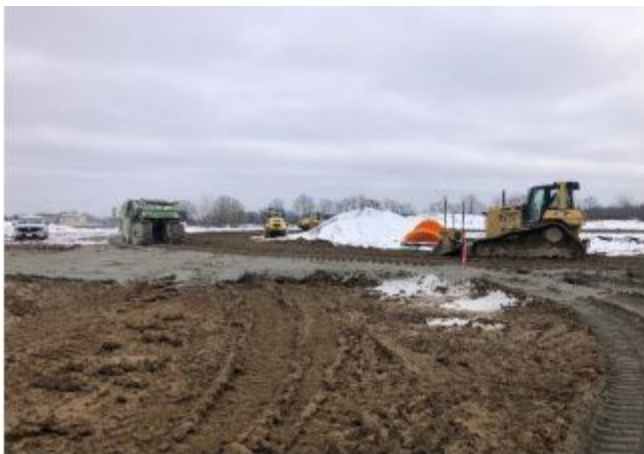
01.08.24 - Cement Stabilization and Grading at Track
