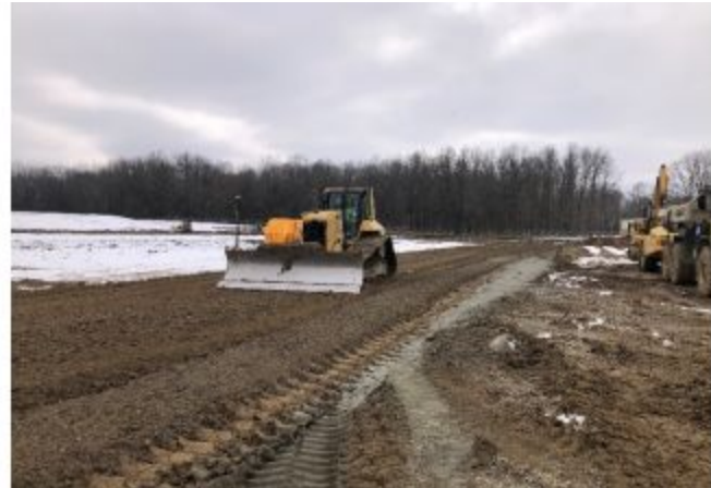
01.08.24 - Cement Stabilization and Grading at Track
