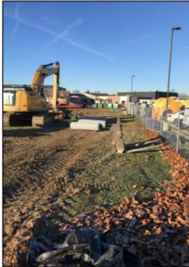
12.14.23 - Storm Sewer Pipe & Structures
