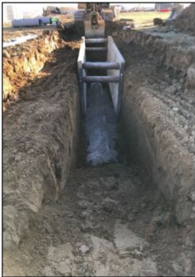
12.14.23 - Storm Sewer Pipe & Structures
