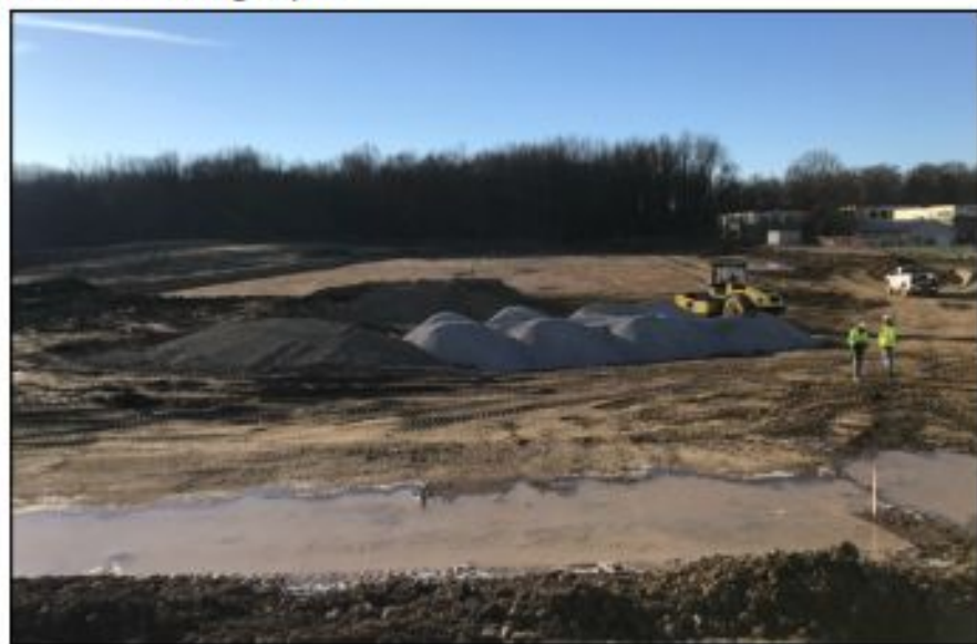
12.14.23 - Rough Grading of Synthetic Turf Field
