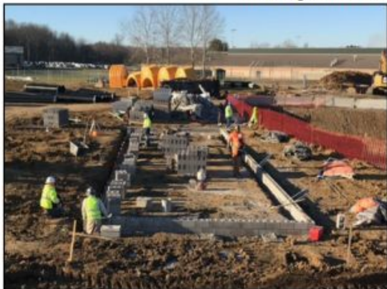
12.14.23 - Masonry Foundation Block at Concession Stand
