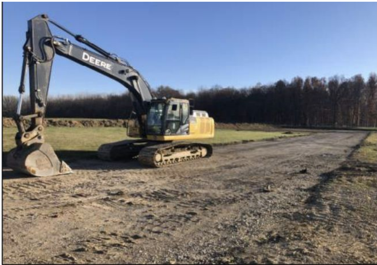
11.15.23 - Demolition of Track complete
