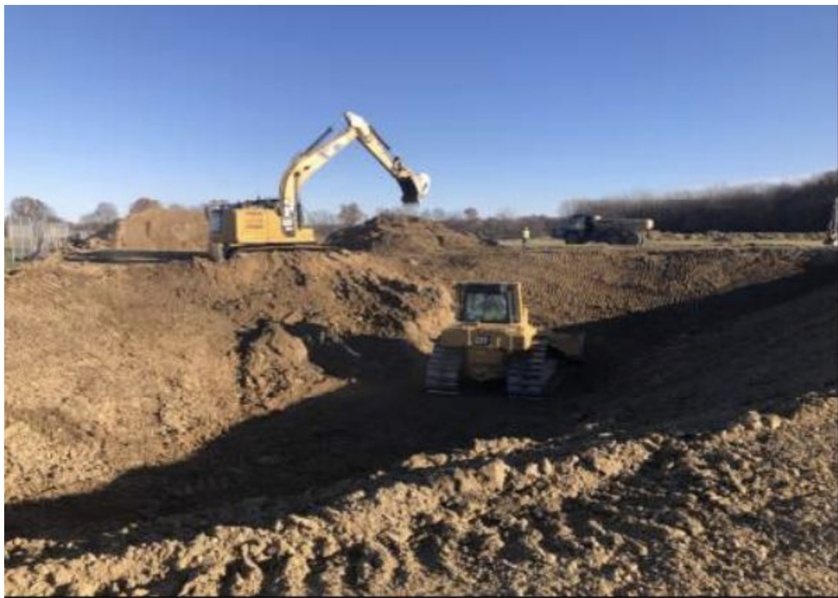
11.15.23 - Excavation of Temporary Sediment Basin
