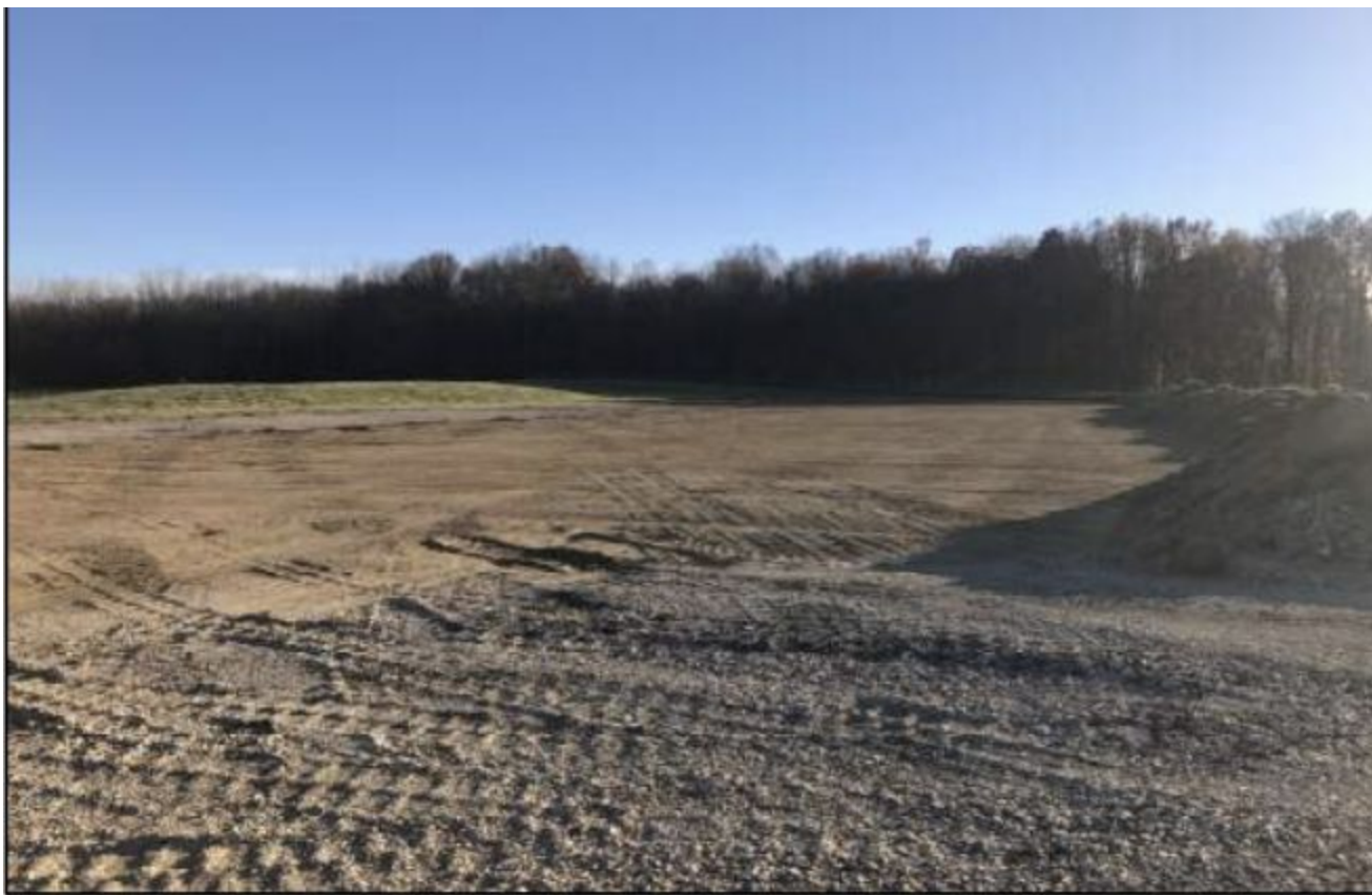
11.15.23 - East half of field topsoil stripped
