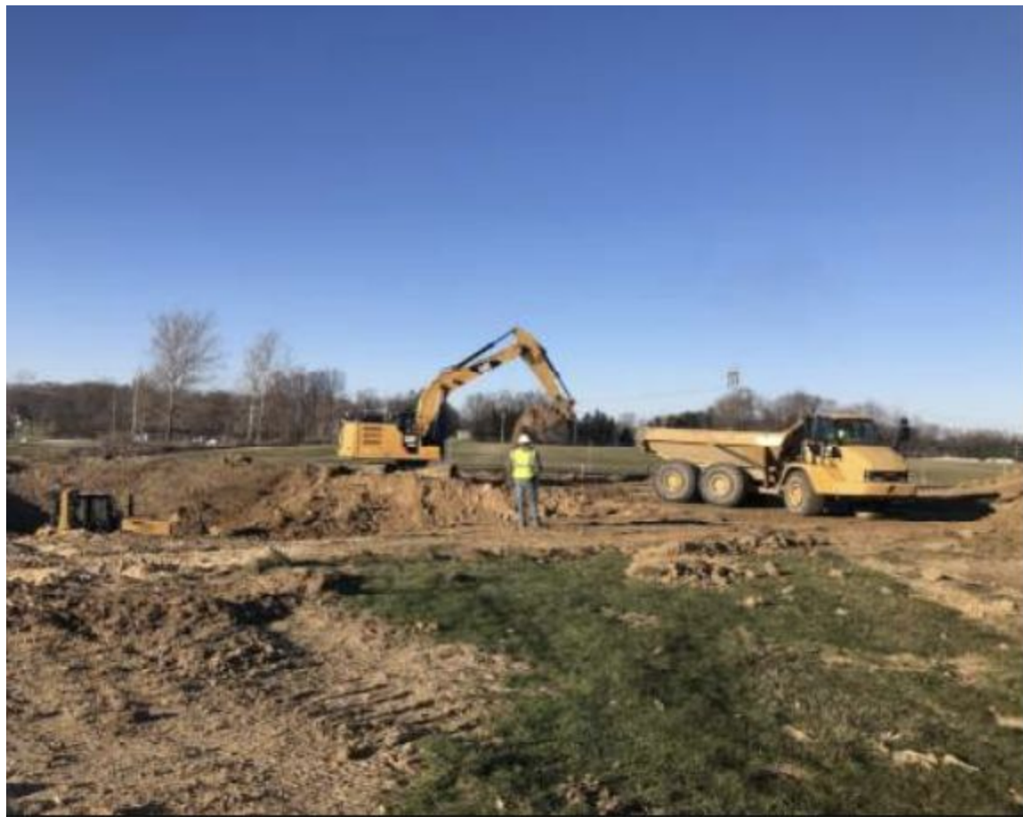
11.15.23 - Excavation of Temporary Sediment Basin
