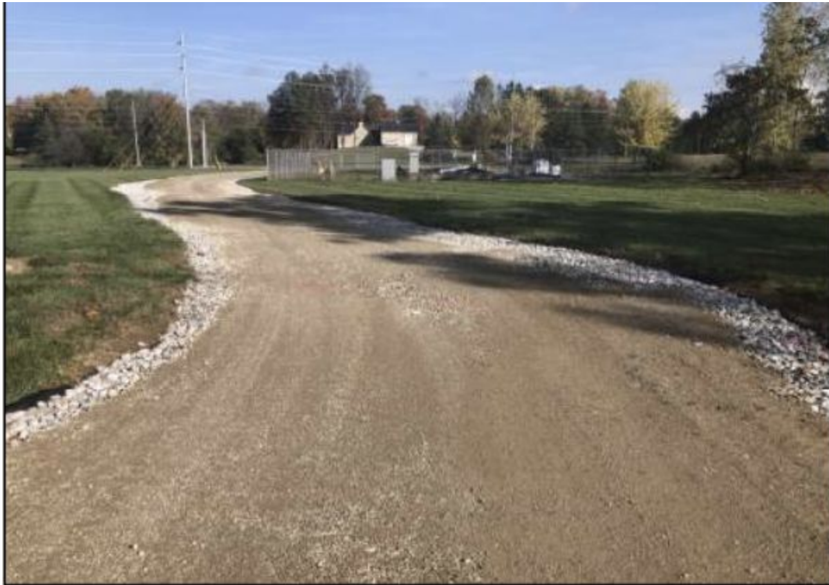
10.18.23 - Temporary Construction Drive installed
