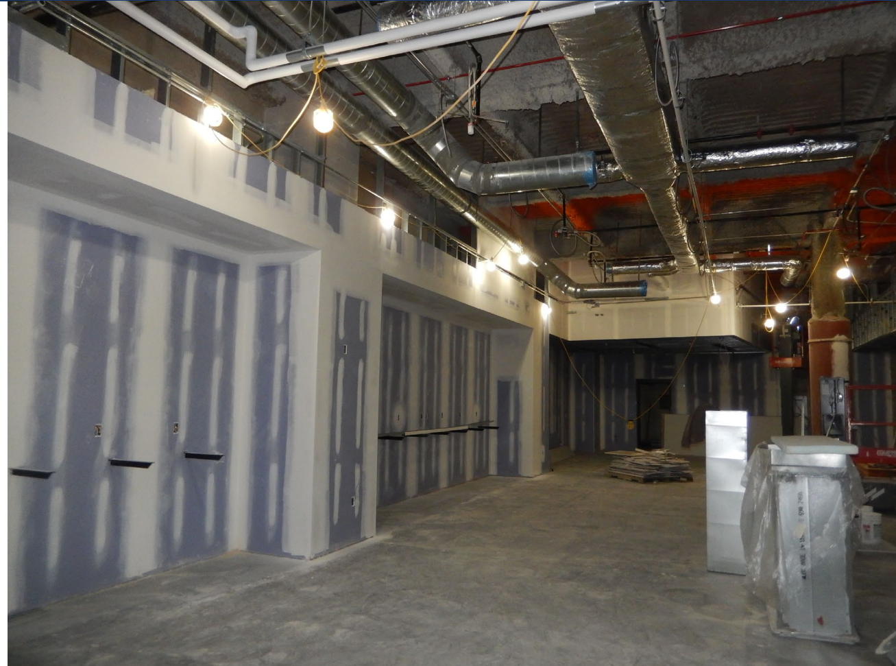
Gypsum board at Media Center
