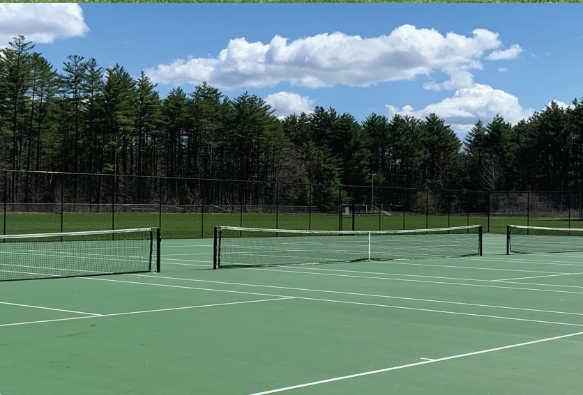
Construction of four competition tennis courts on Howe Street offer students and faculty alike more opportunities to play and compete.
