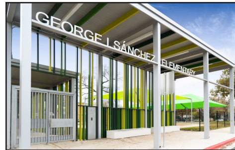
Sanchez Elementary School - Austin, TX
