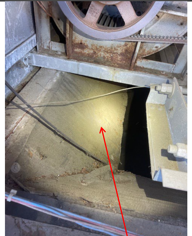
Photo 4: View of ACU1 servicing library. Accumulated dirt and suspect mold growth on damaged/frayed interior duct liner at vertical supply duct.
