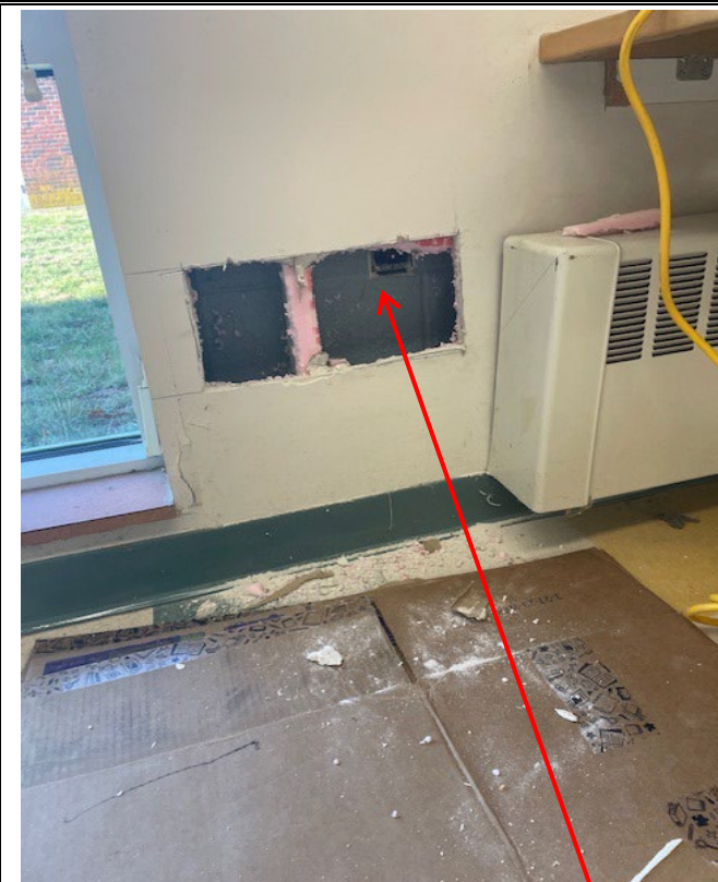
Photo 3: View of classroom 140 at perimeter wall. No suspect mold growth within wall cavity. Original block wall outlet allows outside air leakage to enter wall cavity.
