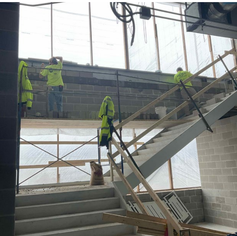
TWO-STORY ACADEMIC AREA STAIRWAY
