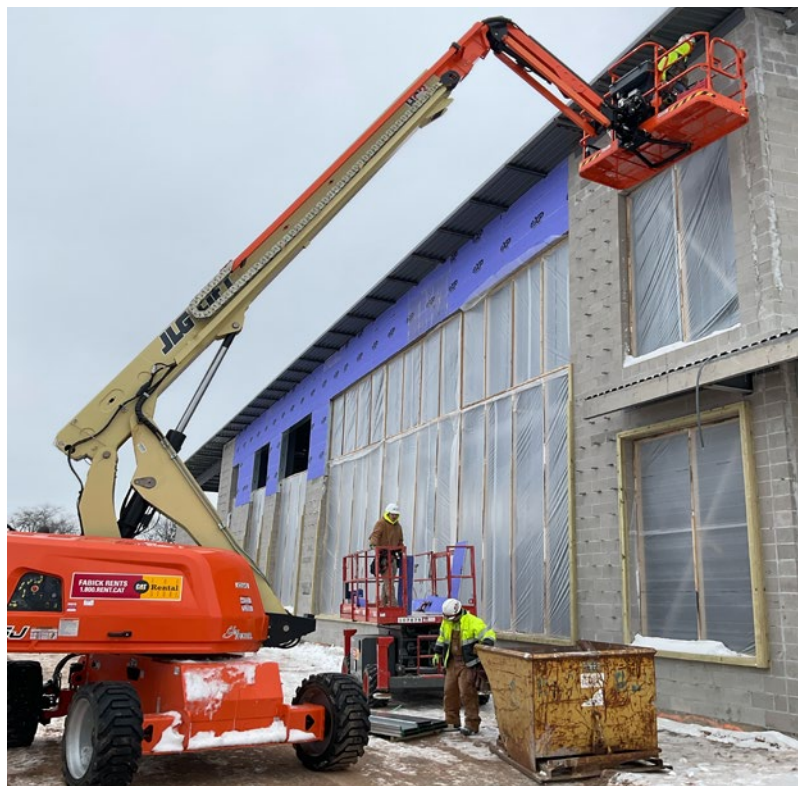
EAST EXTERIOR FACING LAKE WINNEBAGO
