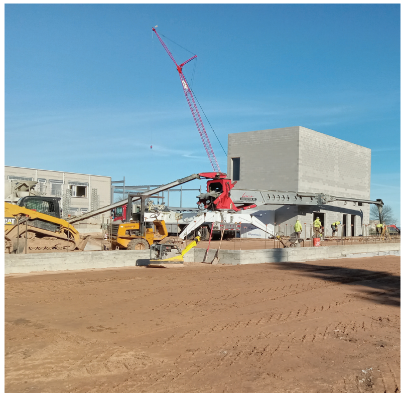
CONCRETE FOOTINGS BEING PLACED
