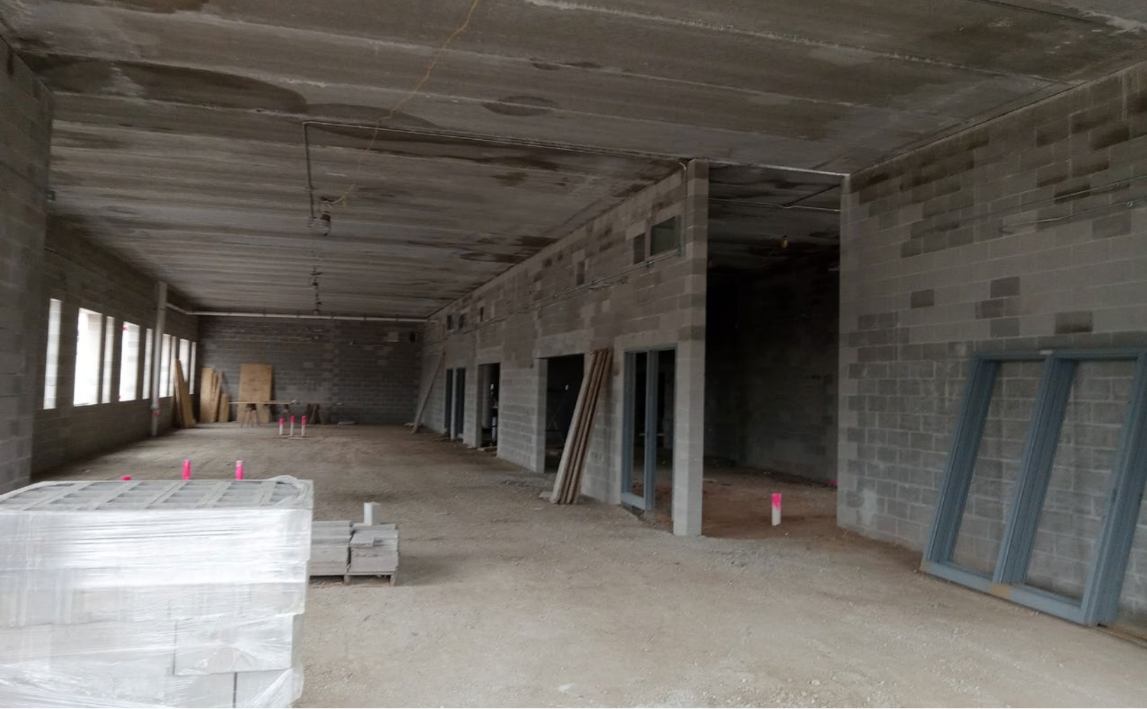
CLASSROOM AREAS BEFORE CONCRETE FLOORS AND DIVIDING WALLS
