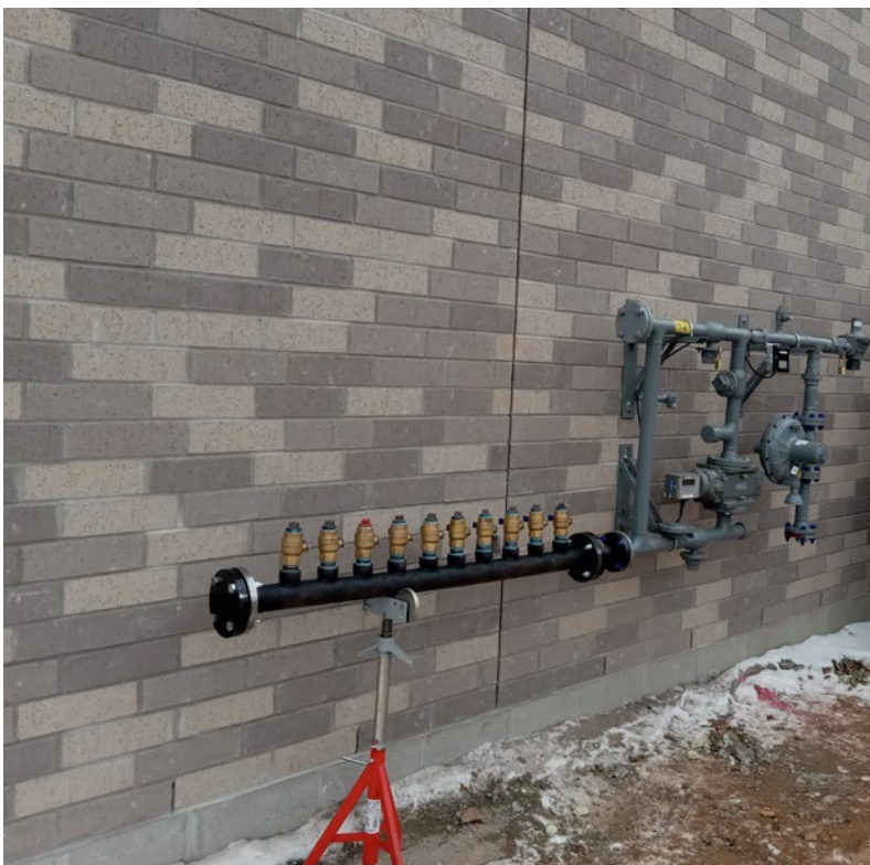
EXTERIOR BRICK INSTALLED ON THE NORTH
