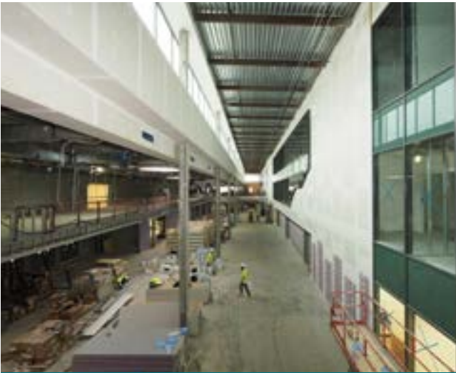
OPENING IN AUGUST 2021! New Upper Arlington High School
