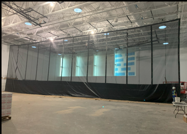
Divider Curtain in Main Gym
