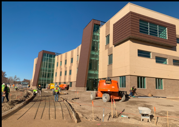
Metal Siding & Site Concrete Prep
