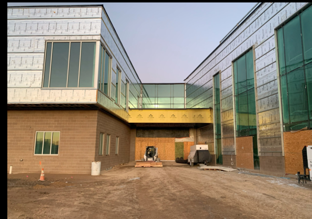
Exterior Glazing and Insulation
