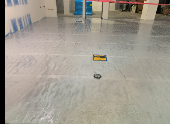
Floor Prep for Terrazzo
