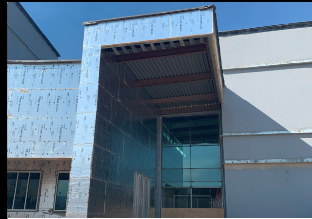
Exterior Glazing and Insulation
