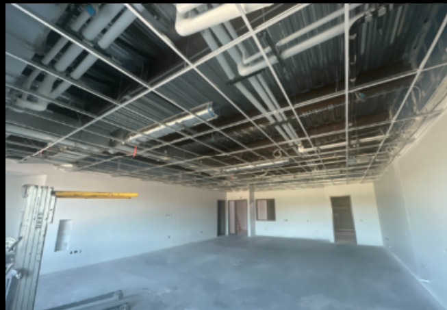
Paint & Ceiling Grid
