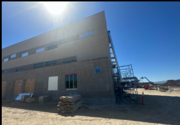
Brick Veneer at Classroom Wing
