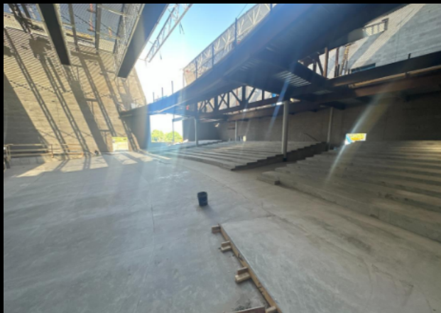
Slab on Grade in Auditorium
