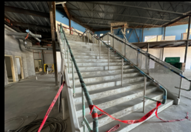
Stairs Installed and Poured
