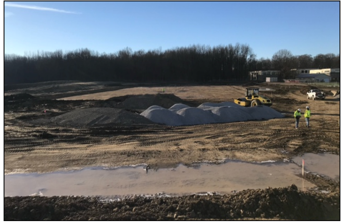
12.14.23 - Rough Grading of Synthetic Turf Field
