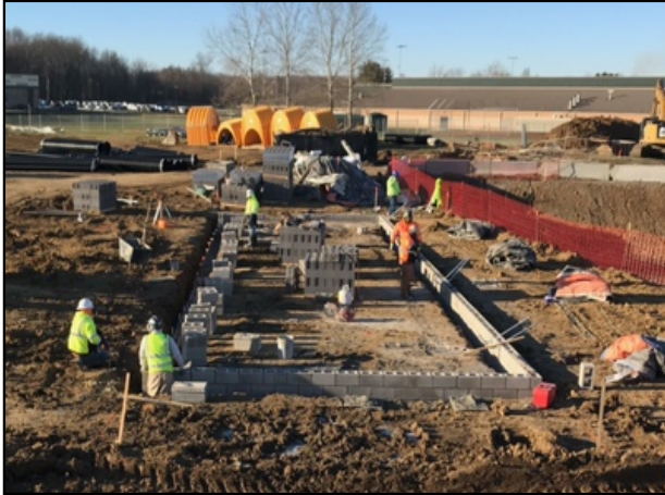
12.14.23 - Masonry Foundation Block at Concession Stand
