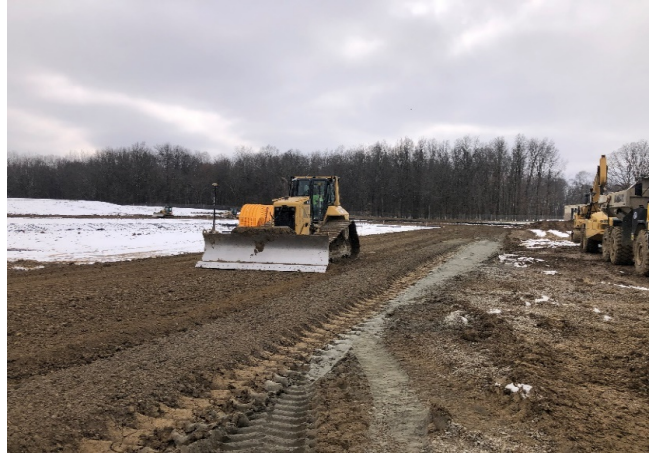
01.08.24 - Cement Stabilization and Grading at Track
