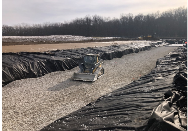
01.05.24 - Excavation for Storm Tech Chambers at Turf Field
