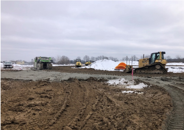
01.08.24 - Cement Stabilization and Grading at Track
