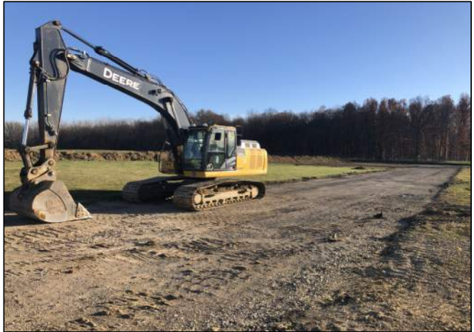
11.15.23 - Demolition of Track complete
