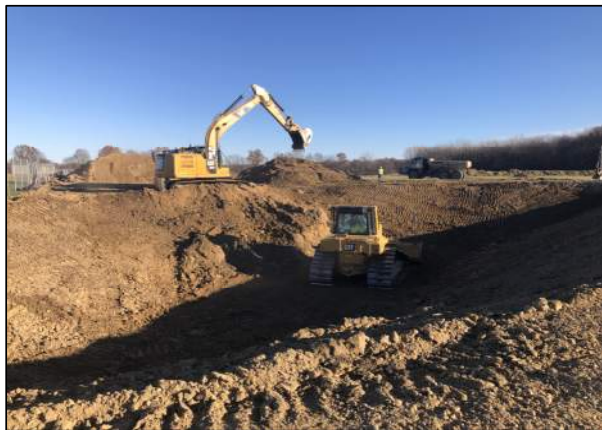
11.15.23 - Excavation of Temporary Sediment Basin
