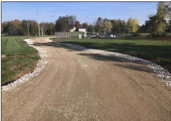
10.18.23 - Temporary Construction Drive installed
