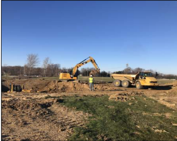
11.15.23 - Excavation of Temporary Sediment Basin
