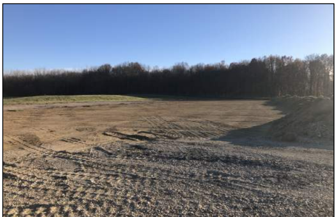
11.15.23 - East half of field topsoil stripped
