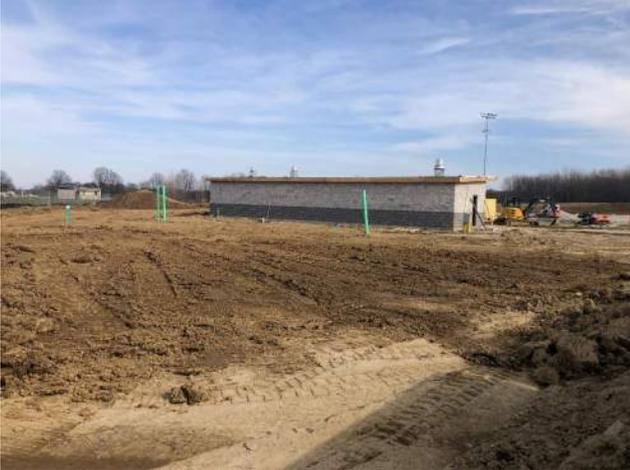
03.12.24 - Temporary Sediment Basin Backfilled
