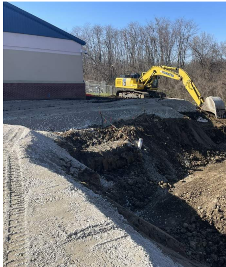
EPiC Elementary - Building Pad
