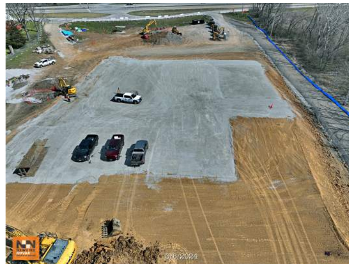
Overall Site/Building Pad
