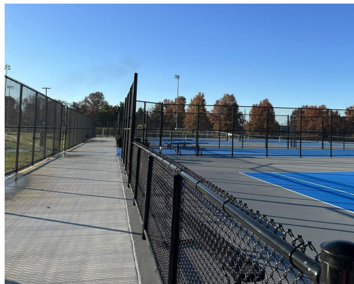
East Concourse Looking South
