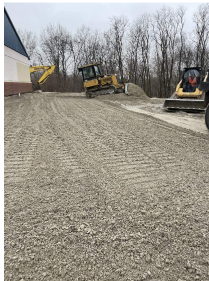
EPiC Elementary - Building Pad
