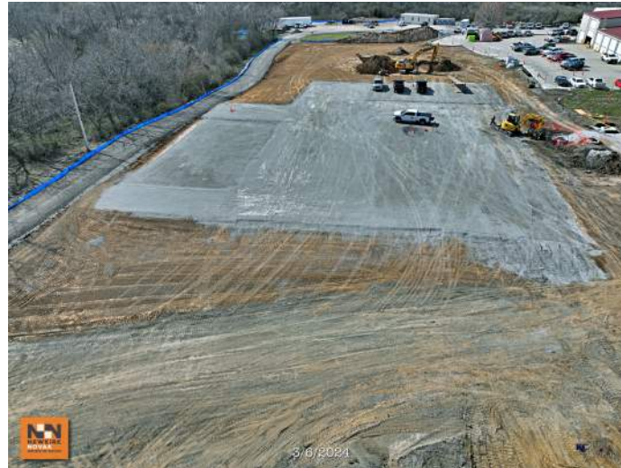
Overall Site/Building Pad
