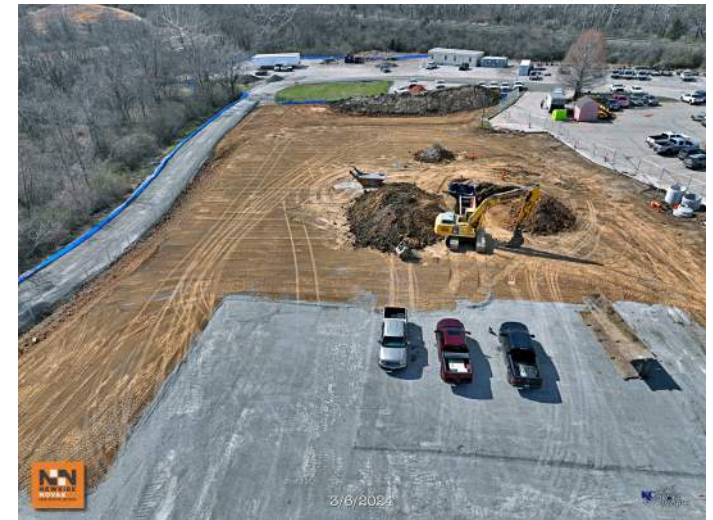
Overall Site/Building Pad
