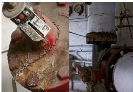
Replace heating and water valves at CRS
