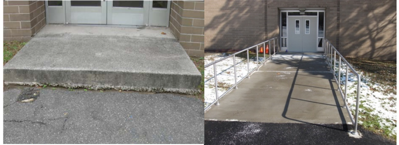
Replaced deteriorated sidewalks and added handicap ramp in rear of AMS
