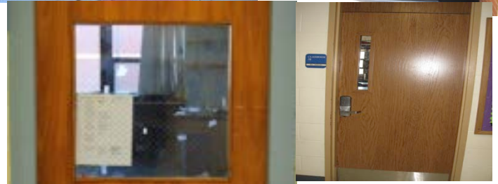
Before and After: New interior and exterior doors
