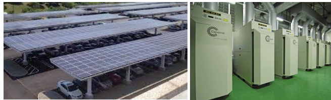
Green Energy: Solar and microturbines
