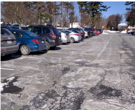
Roadways at AHS and CRS
