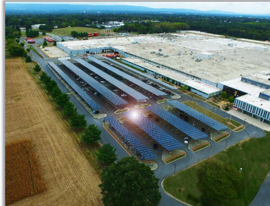
Example of Solar Parking Canopies
