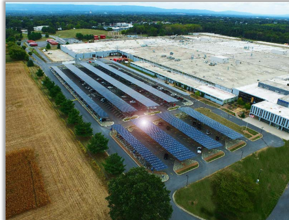
Example of Solar Parking Canopies
