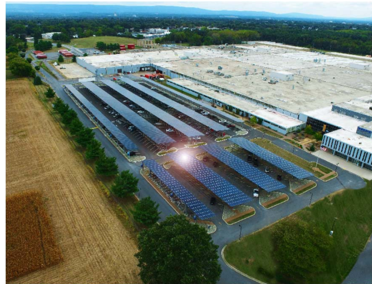
Example of Solar Parking Canopies
