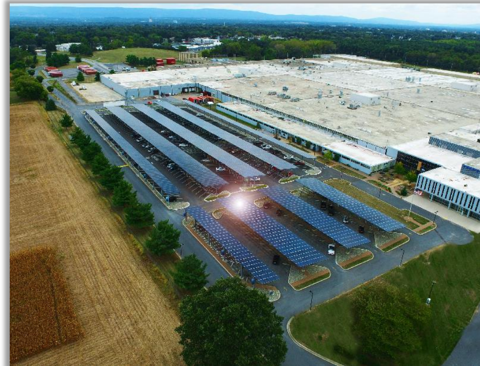
Example of solar parking canopies
