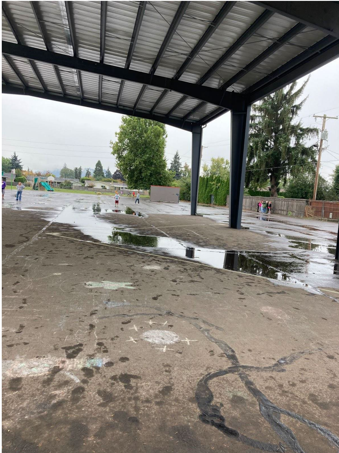
Taken 10/9 at 12:19 pm. The covered area had been totally dry an hour before at 11:20 am. This is not a standing puddle but a stream or water moving down the slope of the blacktop.
