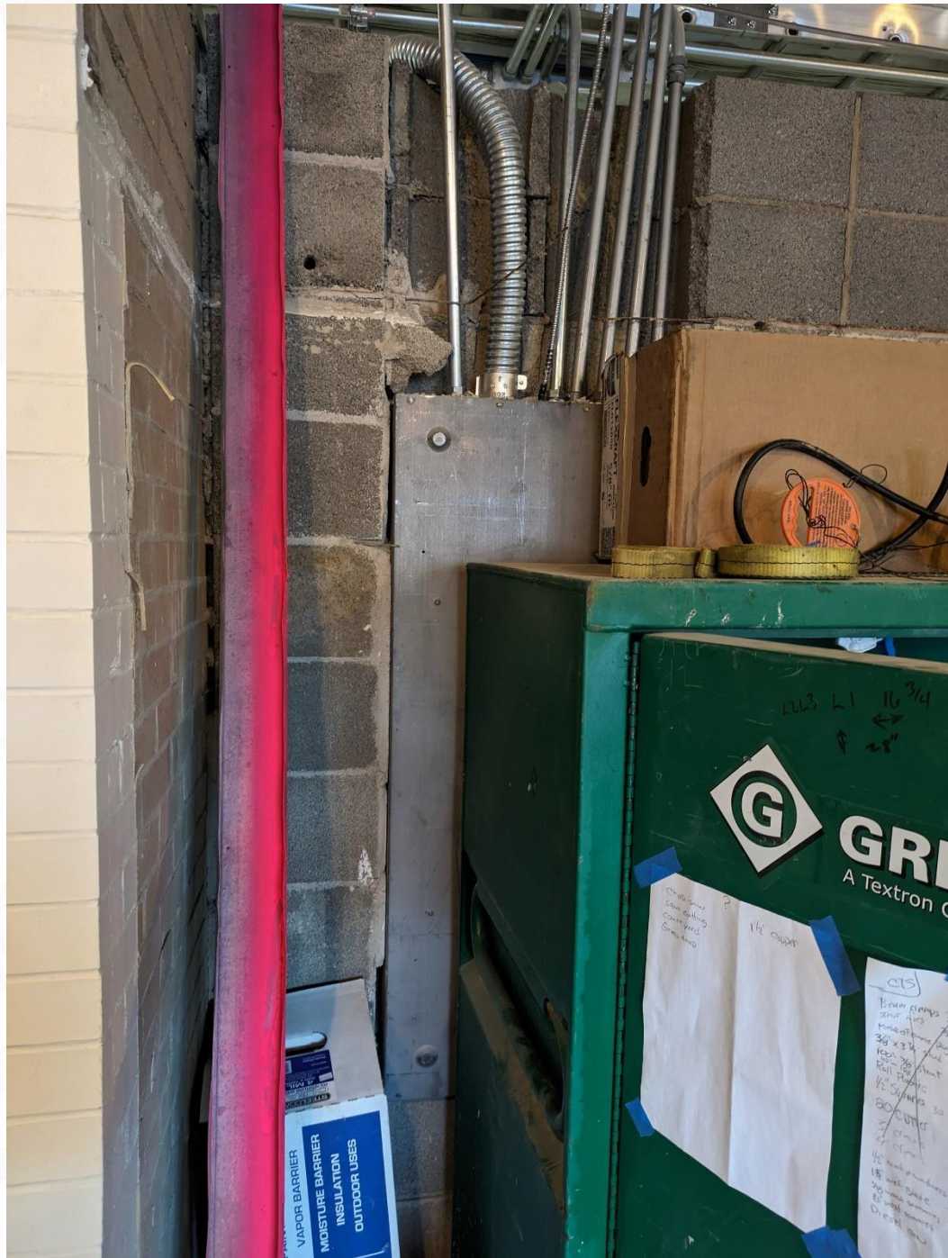
Classroom side of corridor wall. Electrical panel will need to be built out and drywalled over
