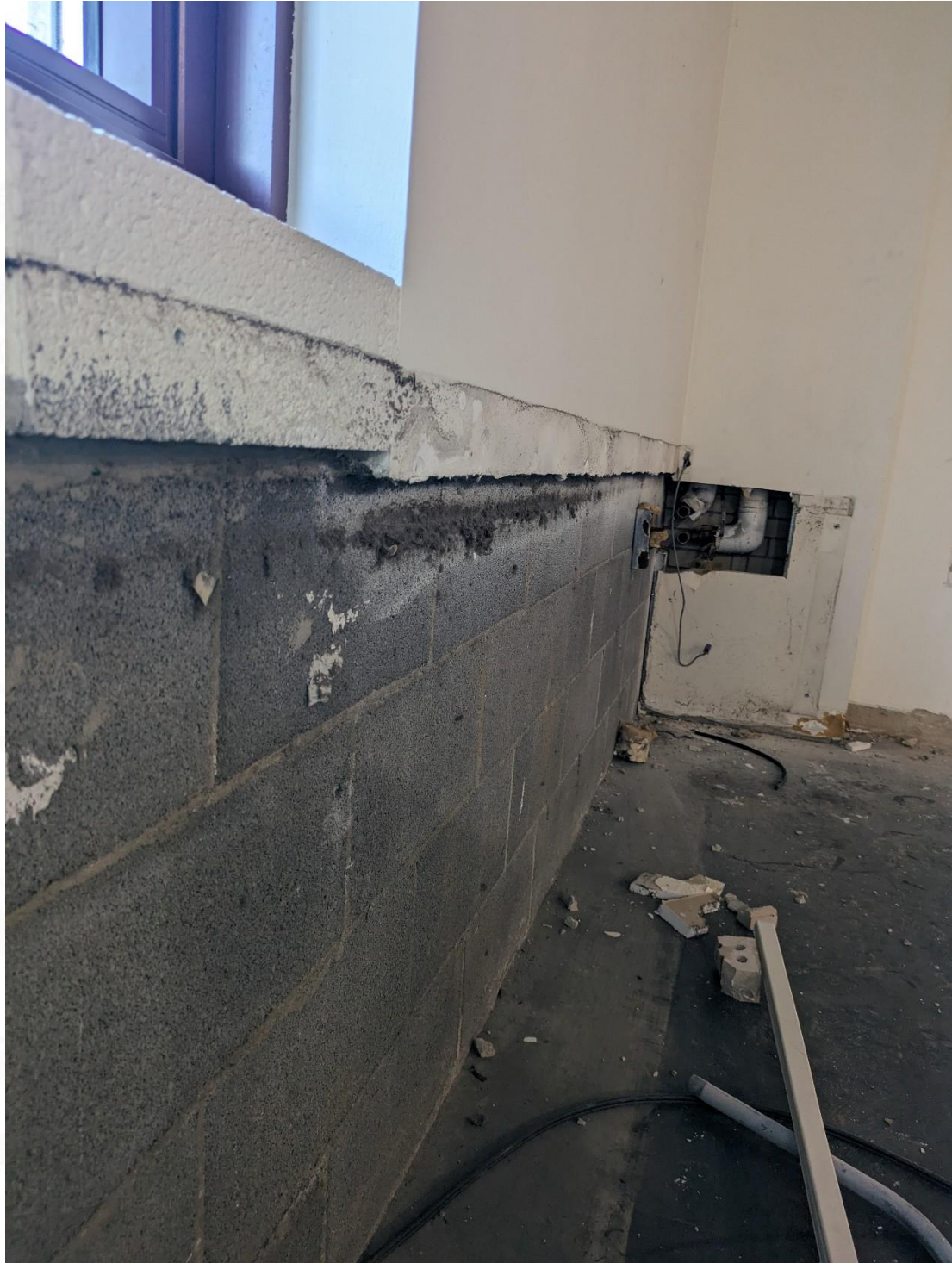
View of uneven plane between existing plaster and block wall. Lower portion will be framed out and drywalled.
