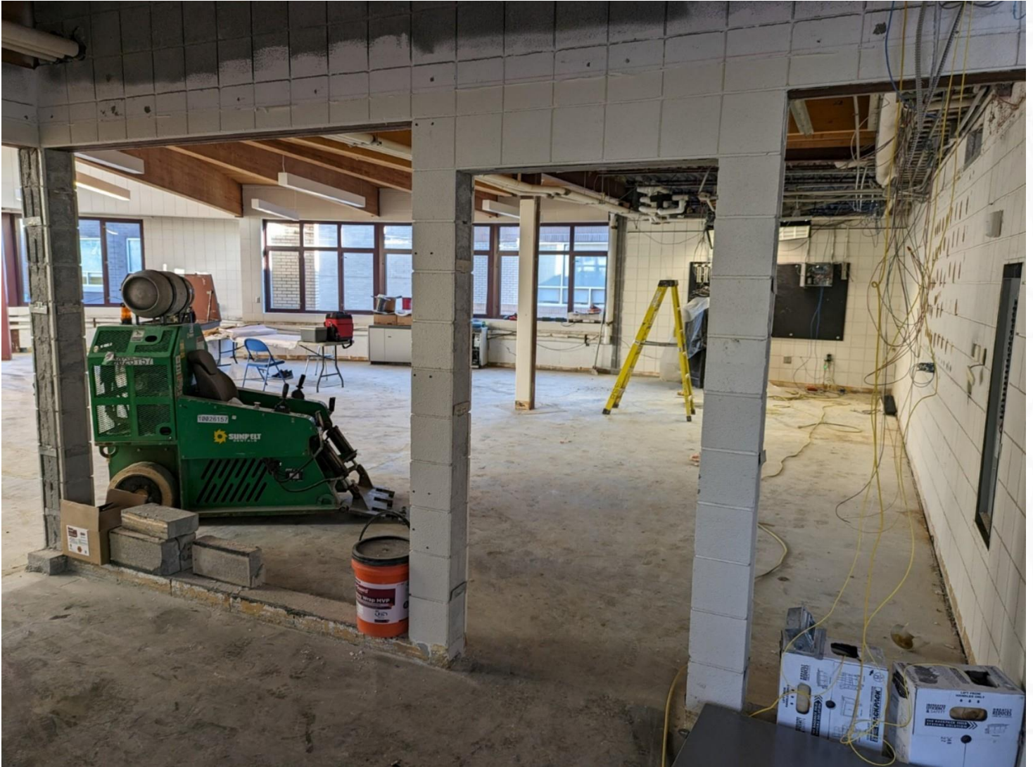
Selective demolition is nearly complete in library
