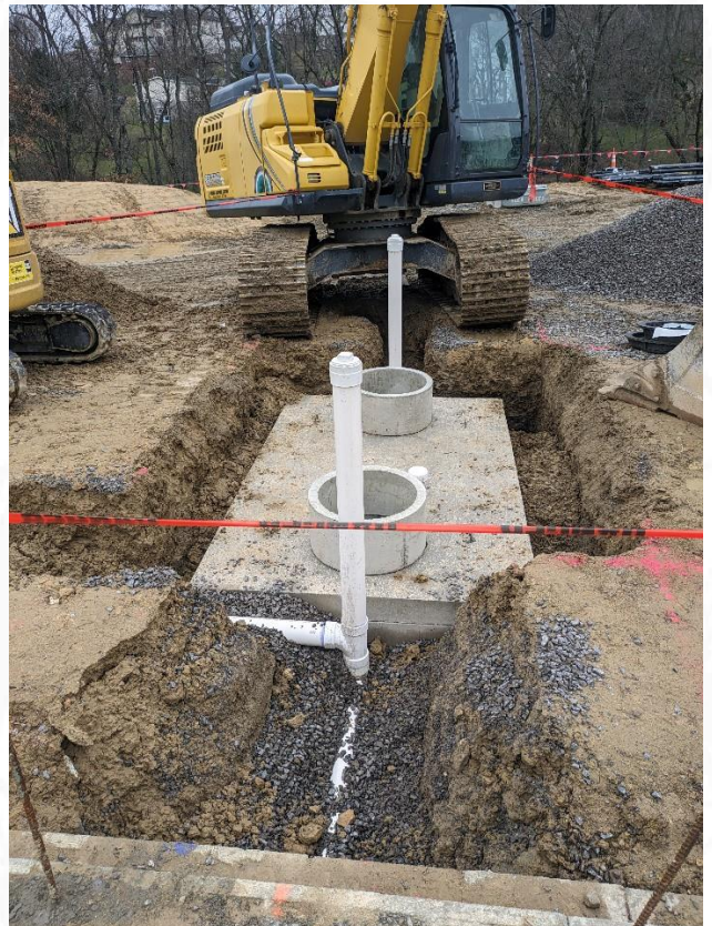
Grease Interceptor for kitchen being installed
