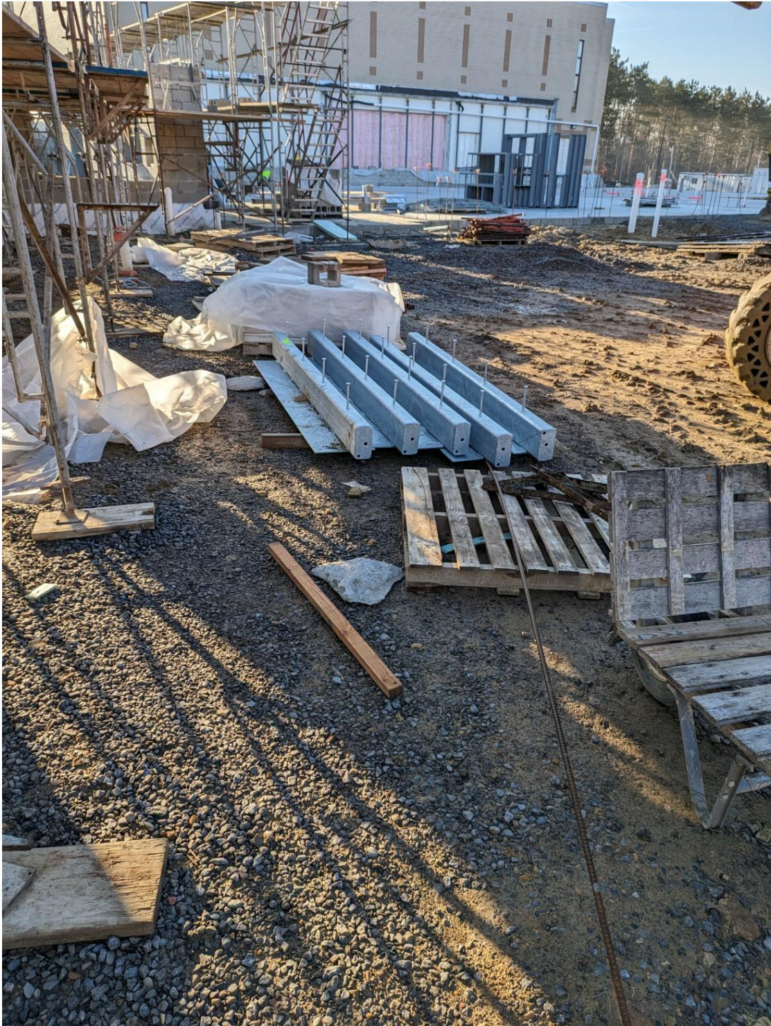
Lintels for exterior windows ready for installation
