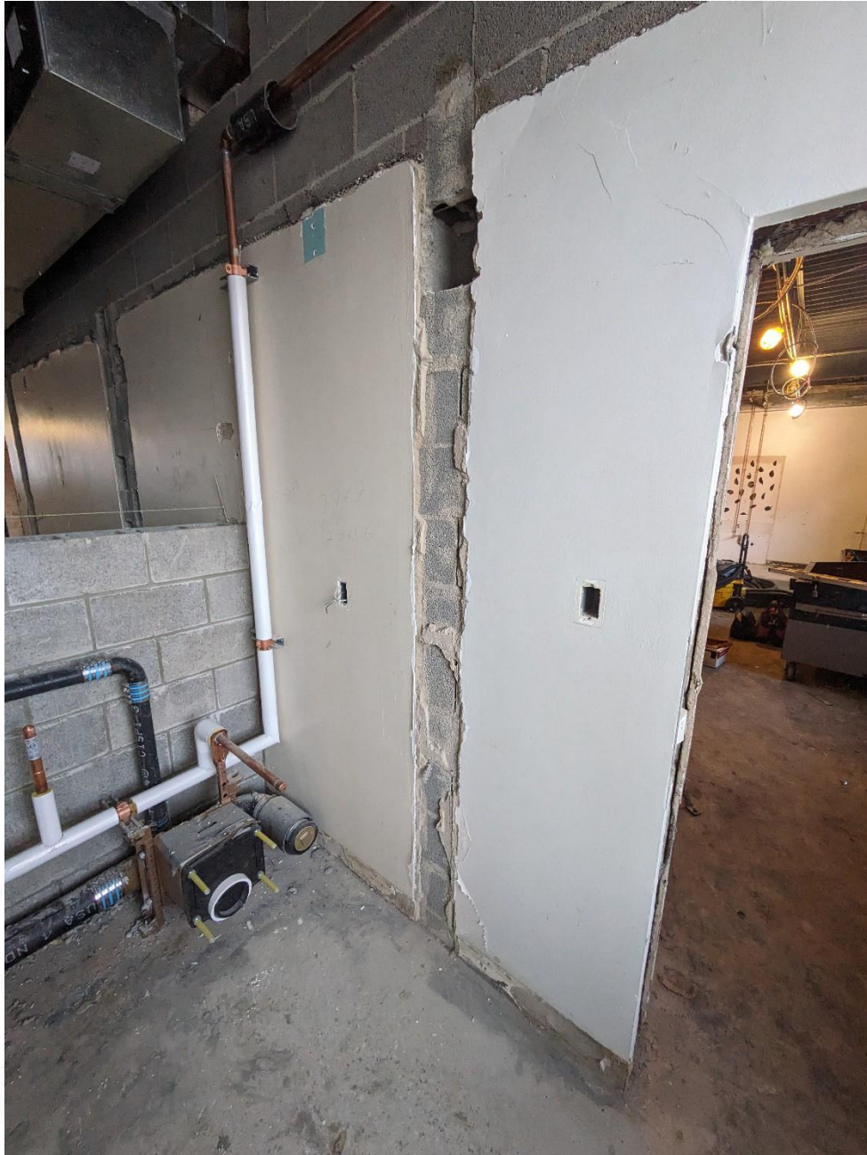
New plumbing chase under construction in restroom for the Emotional Support classroom. Also shows uneven plaster that will be covered over.
