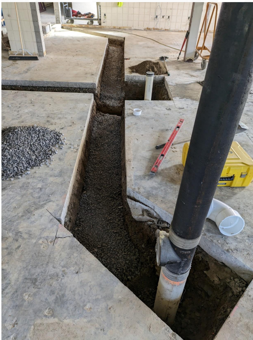
New underground storm and sanitary lines in former office area to be part of new art room
