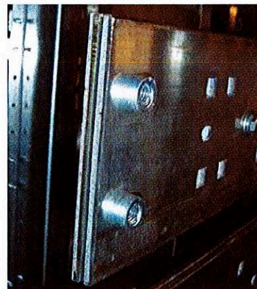
(Picture #4) (Cross Bus Backside do not install on this side) WRONG do not install links on top of captive nuts
