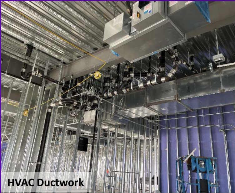
Interior Wall Framing
