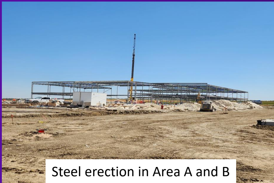
Steel erection in Area A
