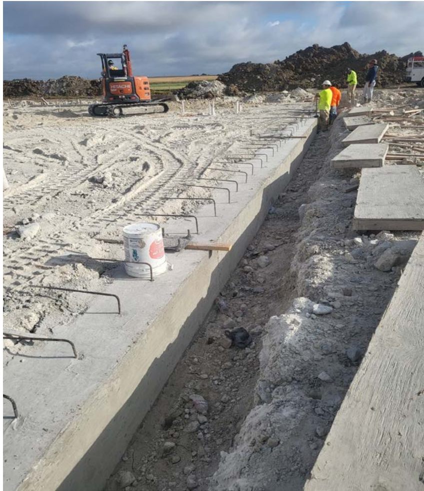
Grade beam installation
