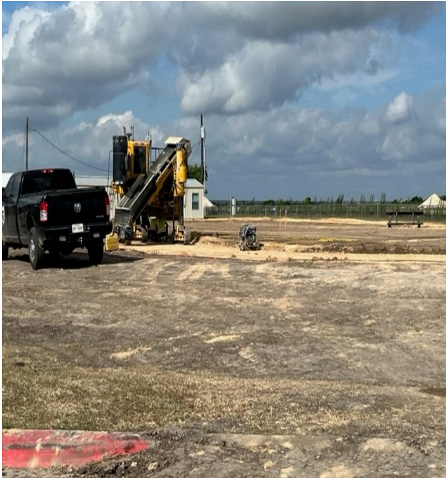
Installing ribbon curbs at Neidig track
