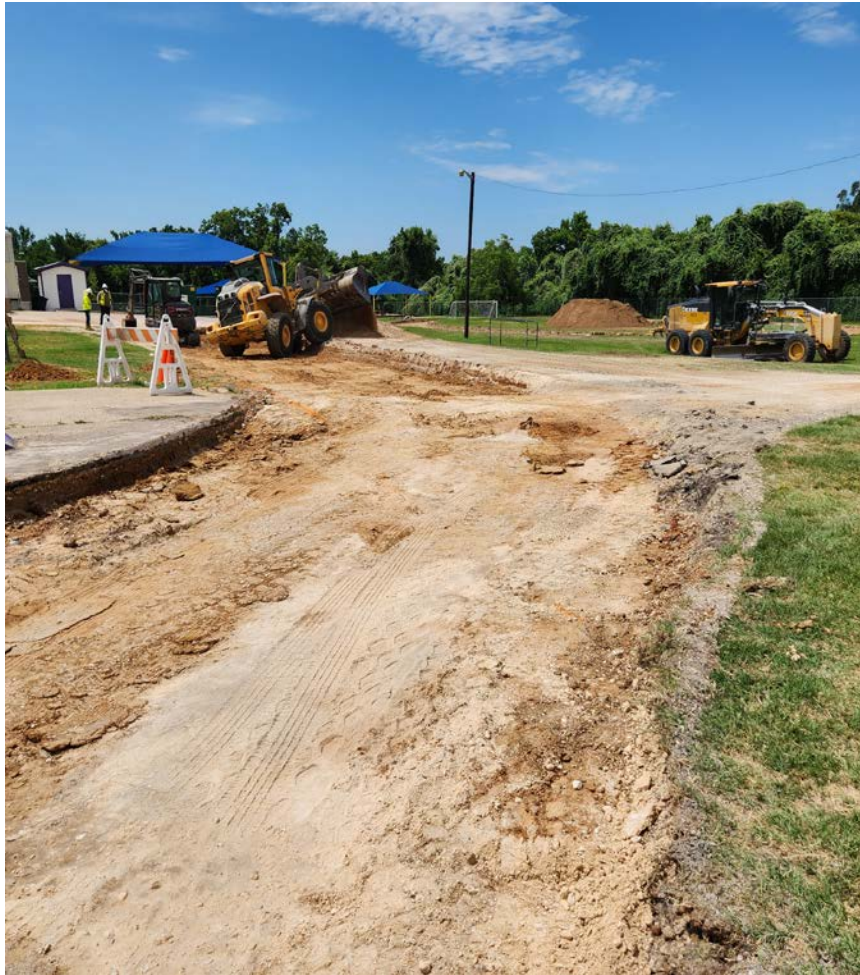
Booker T. Washington paving renovation
