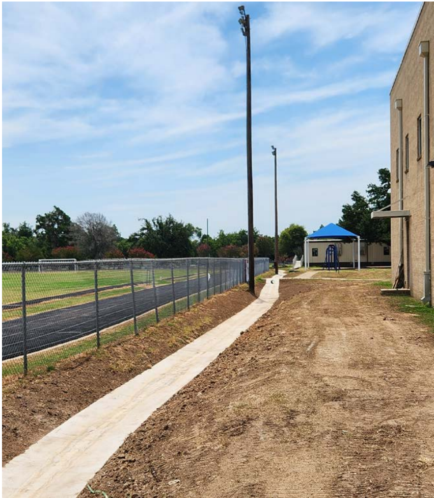
Elgin Elementary drainage improvements
