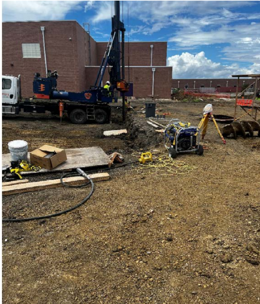
Pier drilling at auditorium
