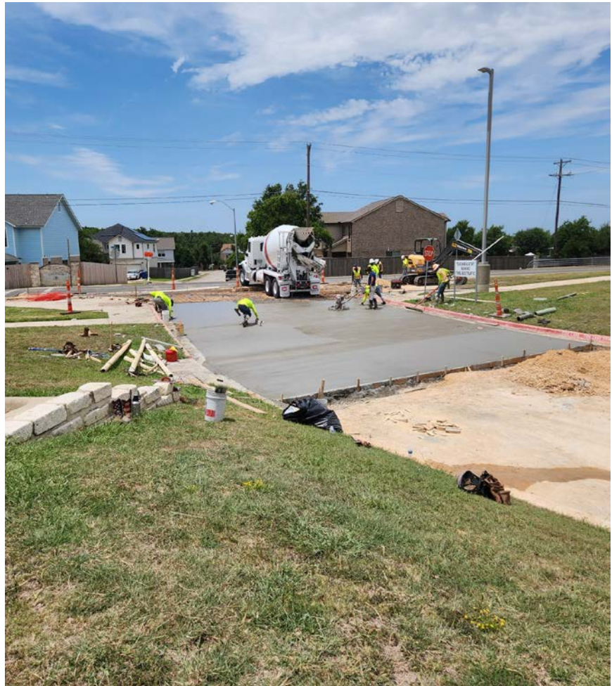
Middle School paving improvements
