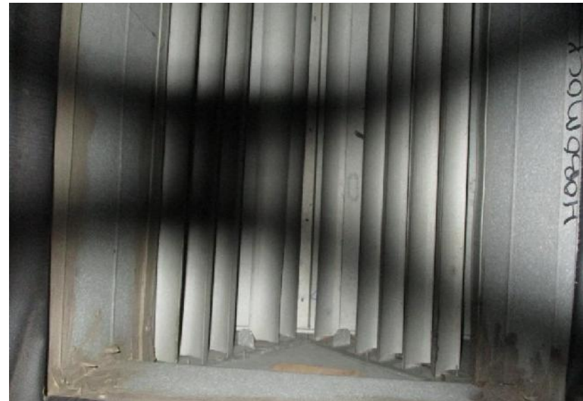
16) Supply air grille with considerable fouling.
