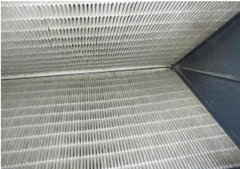
11) Secondary air filter in overall acceptable sanitary condition.
