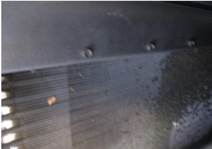
5) Cooling coils with considerable fouling.
