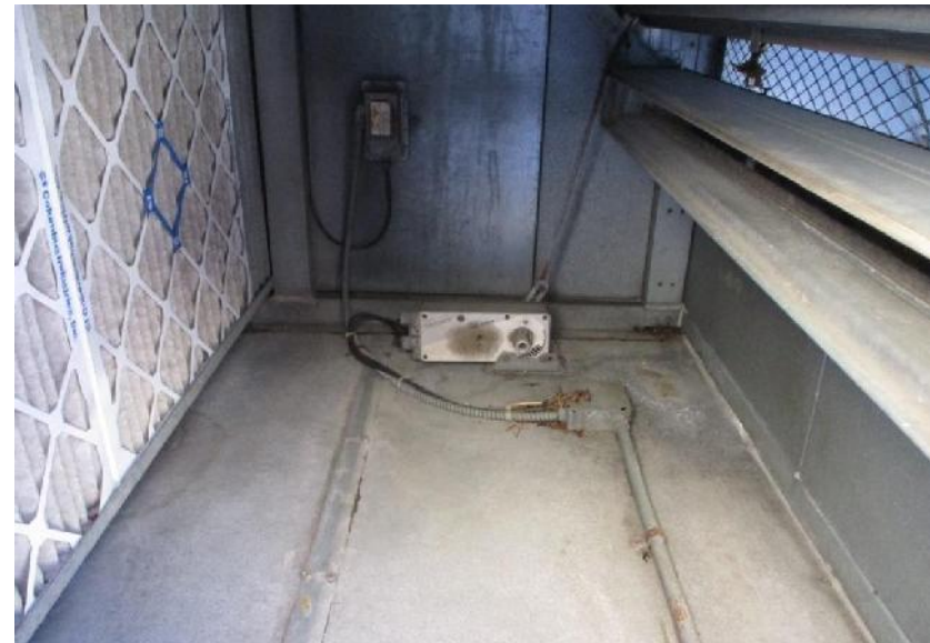
2) Return plenum with considerable fouling.
