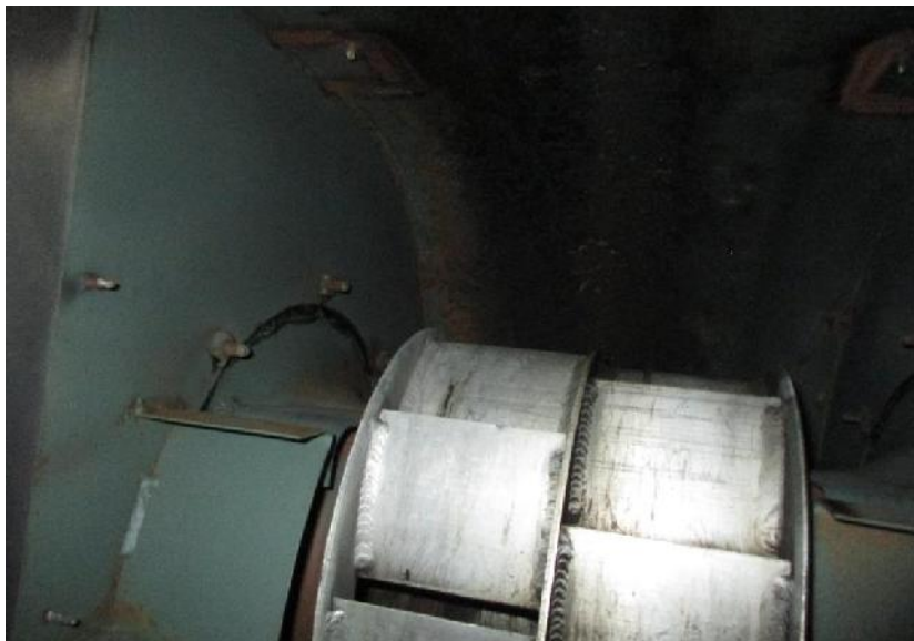
7) Blower wheel in marginal sanitary condition.
