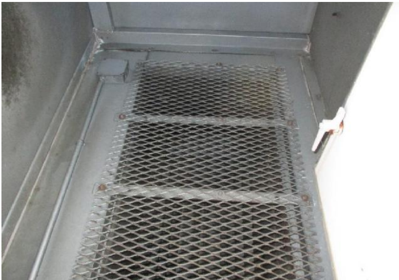
15) Supply air plenum in good sanitary condition.
