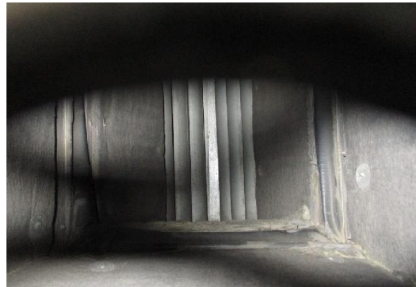
8) Supply air duct in marginal sanitary condition.
