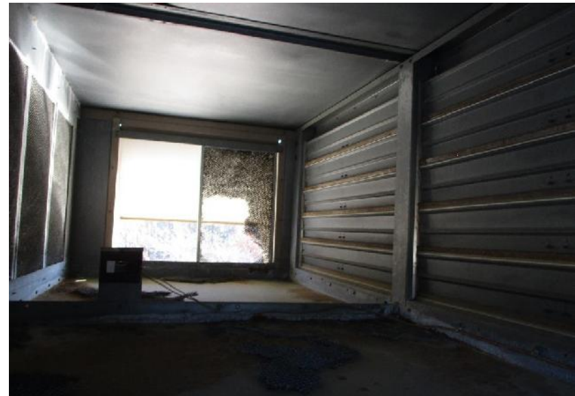
18) Return plenum with considerable fouling and deteriorated O/A filtration.
