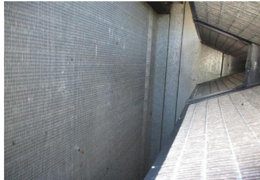
12) Cooling coil in overall acceptable sanitary condition.
