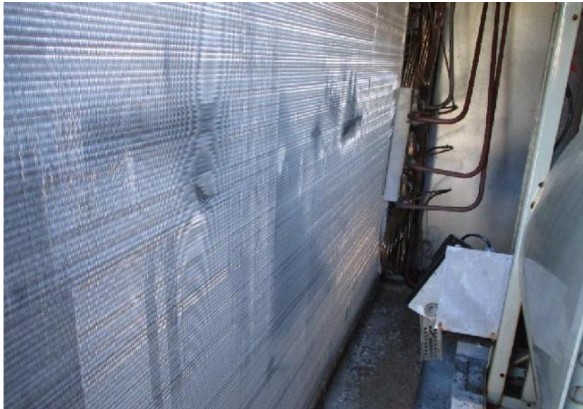
21) Downstream side of cooling coil in good sanitary condition.
