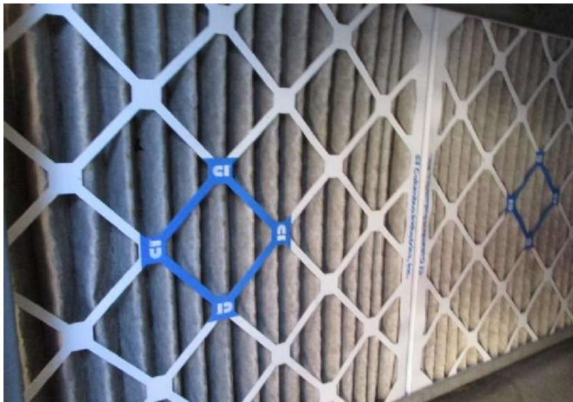
3) Air filters in marginal sanitary condition.
