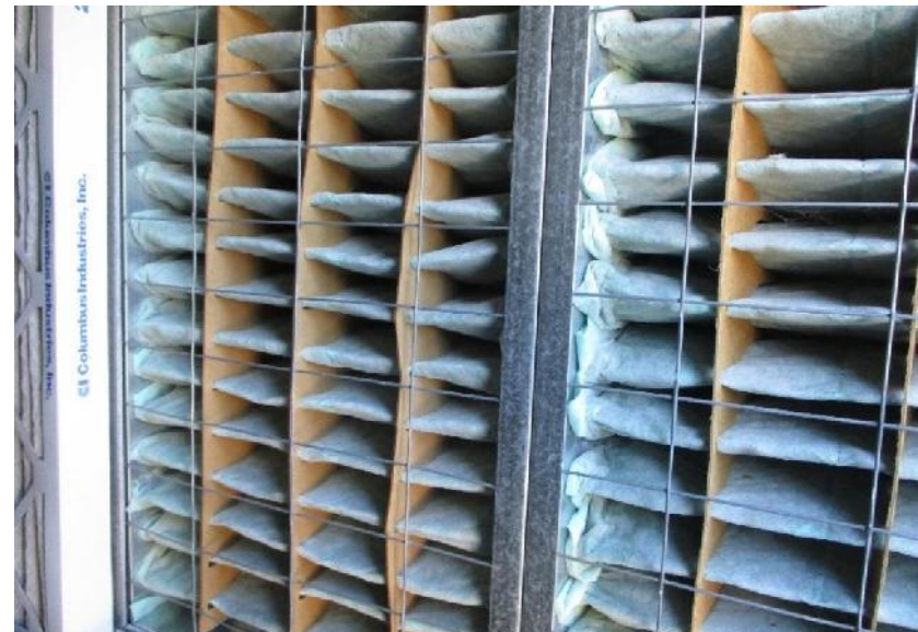
20) Secondary air filters in good sanitary condition.
