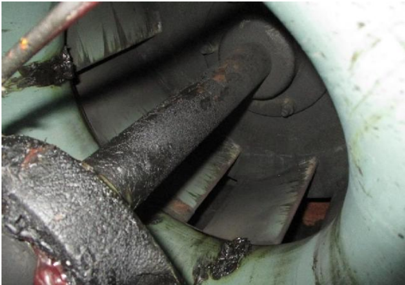
13) Blower housing with considerable fouling.
