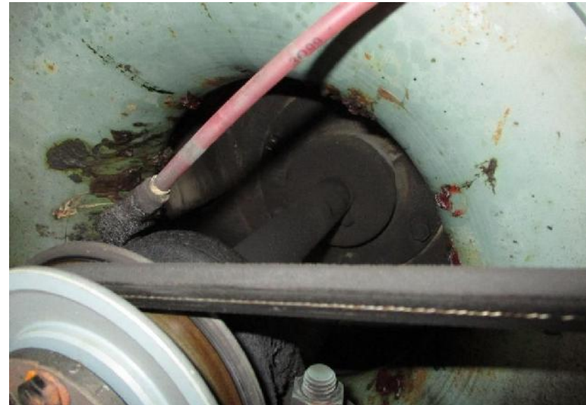
6) Blower housing with considerable fouling.
