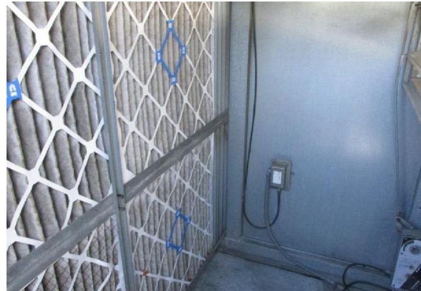
10) Return air plenum and air filters in overall acceptable sanitary condition.
