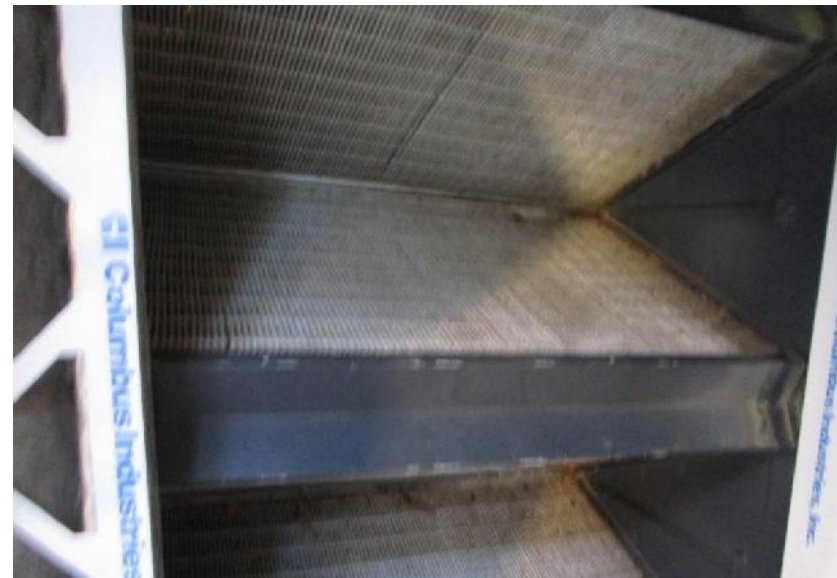
4) Secondary filters with considerable fouling.
