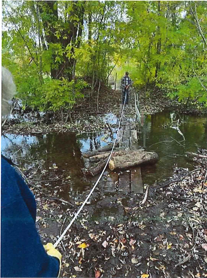
Spur Trail Bridge 1
