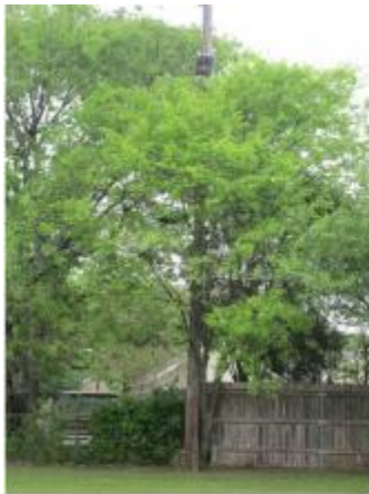
Photo 3 View of pole-mounted transformer on the northern boundary of the site
