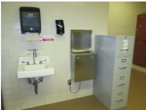
Photo 59 General view of the kitchen area in the cafeteria building
