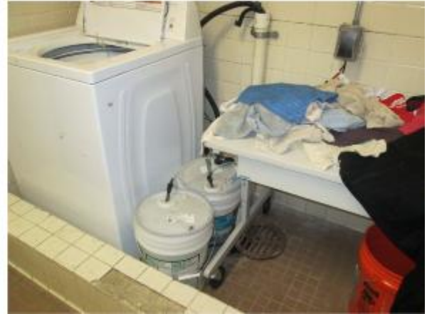
Photo 56 View of laundry area in the cafeteria building
