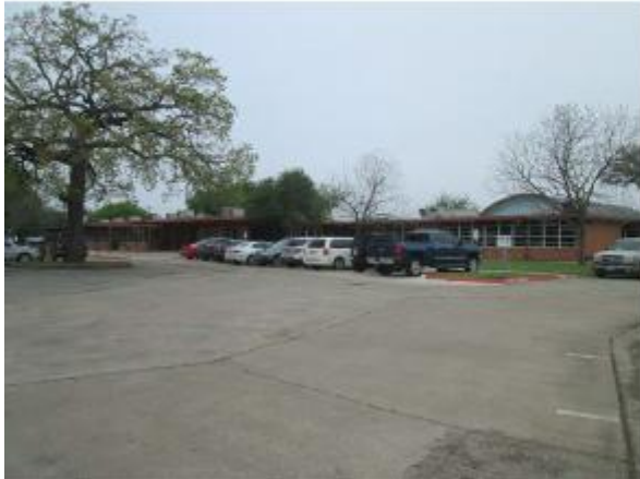
Photo 19 General view of the main building
