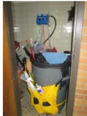
Photo 34 View of janitorial closet in the main building
