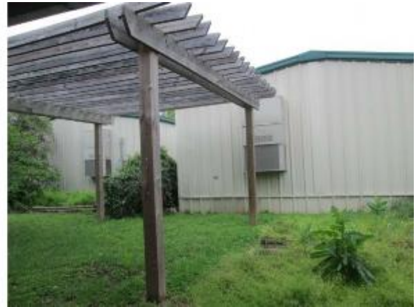
Photo 40 View of the portable buildings
