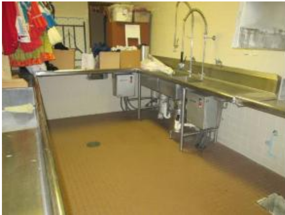
Photo 57 General view of the kitchen area in the cafeteria building
