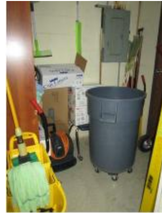
Photo 32 View of janitorial closet in the main building
