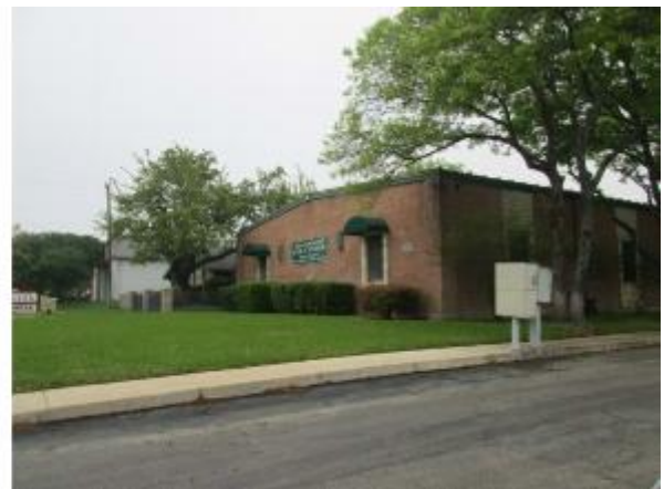
Photo 78 View of the west adjoining properties (San Gabriel Optical & Comfort Keepers Home Care)
