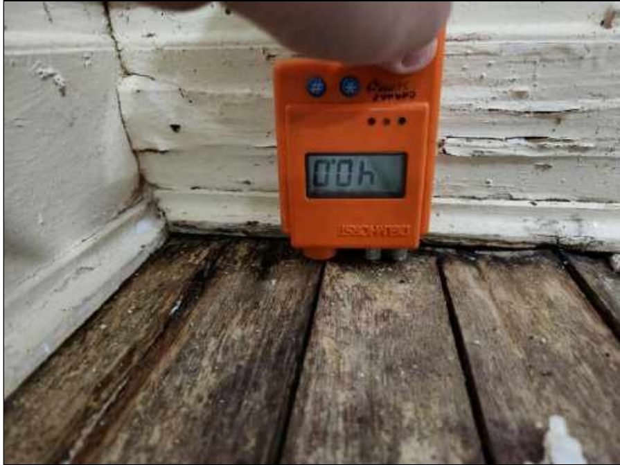
15 - Wet moisture meter reading collected from the stage floor
