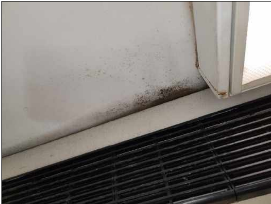
6 - Mold on the plaster ceiling in a classroom in the basement of the original building
