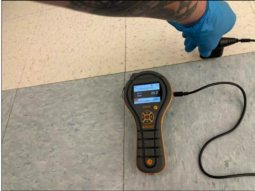
9 - Elevated Moisture Meter Reading From Floor Tile in Room 105
