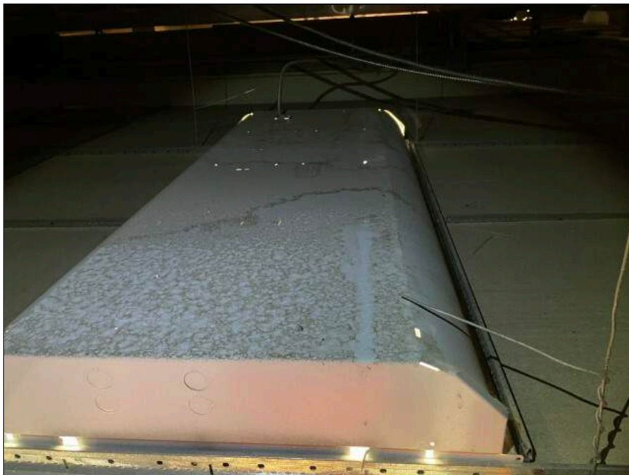
14 - Moisture Staining on a Light Fixture in the NE Corner of the Media Center
