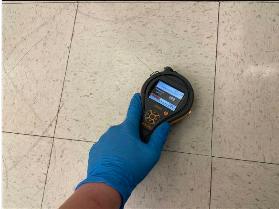
11 - Lower Moisture Meter Reading in the Middle of Room 118 Relative to elevated Reading by the Back Door
