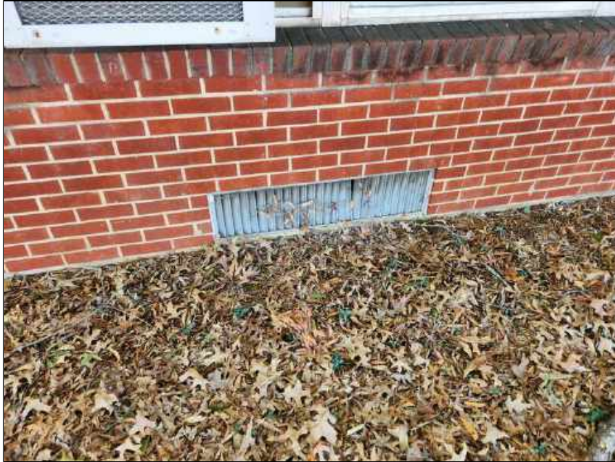
5 - Exterior Grade at the Level of the Fan Coil Intake
