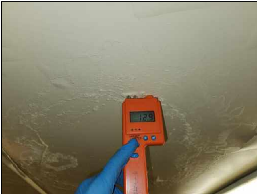
2 - Moisture Meter Indicating the Plaster Ceiling is Dry
