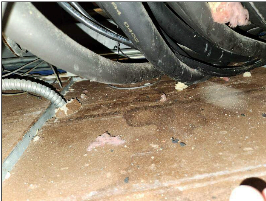
4 - Moisture staining and suspect mold on the back of a ceiling tile in the exterior exit hallway
