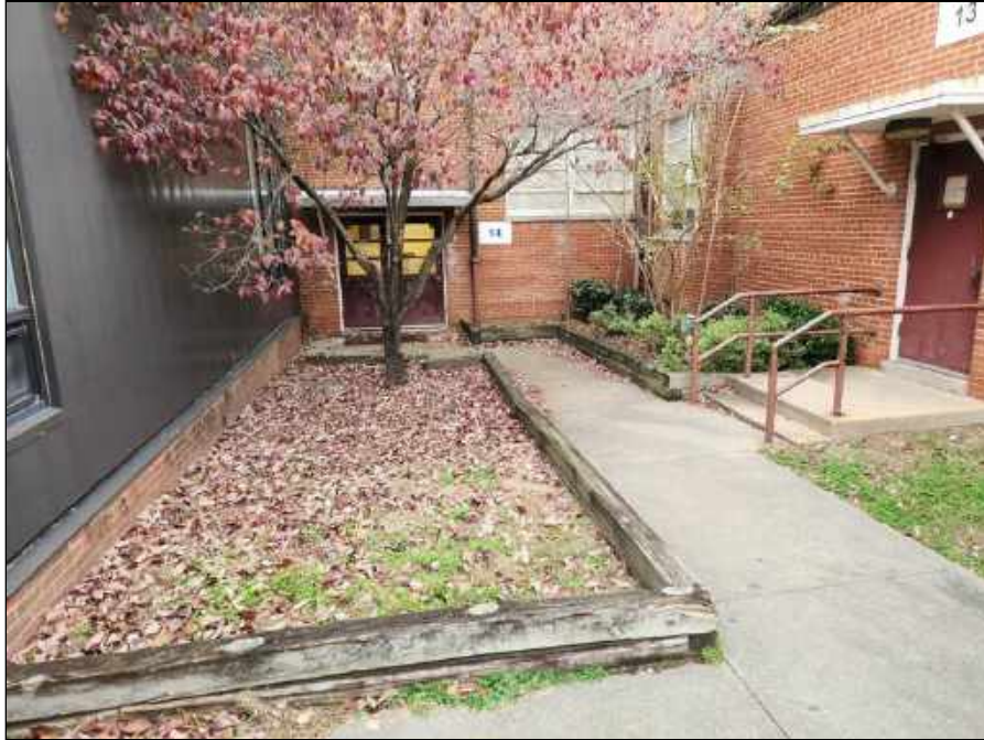
7 - Courtyard between the Activities portion of the building and the Cafeteria
