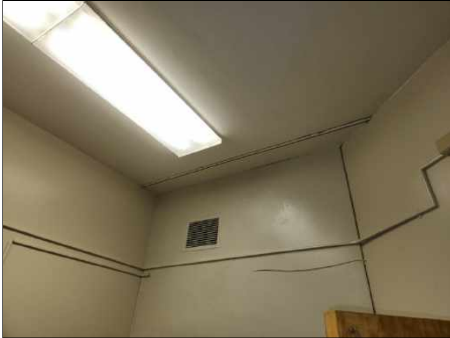
15 - Repaired plaster wall in room 111 observed on 10-30-23
