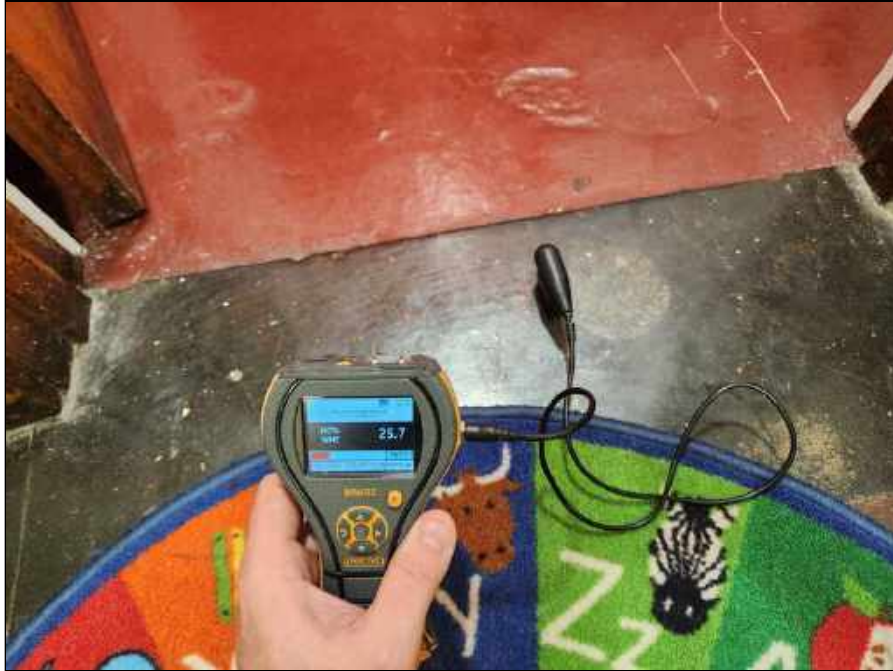
1 - Moisture meter reading collected in the Room 101 bathroom indicating elevated moisture beneath the flooring
