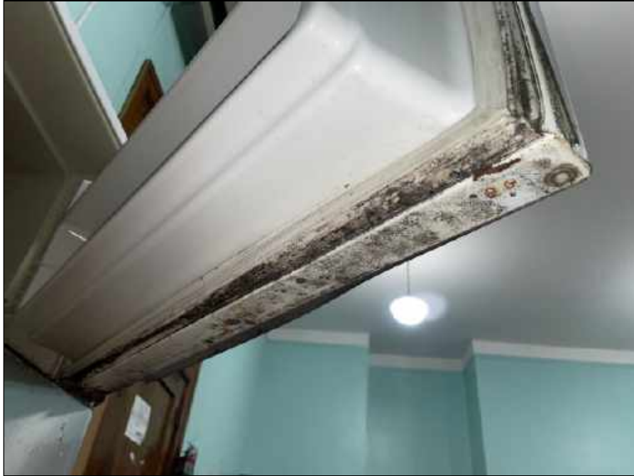
35 - Mold on the refrigerator door in Room 111
