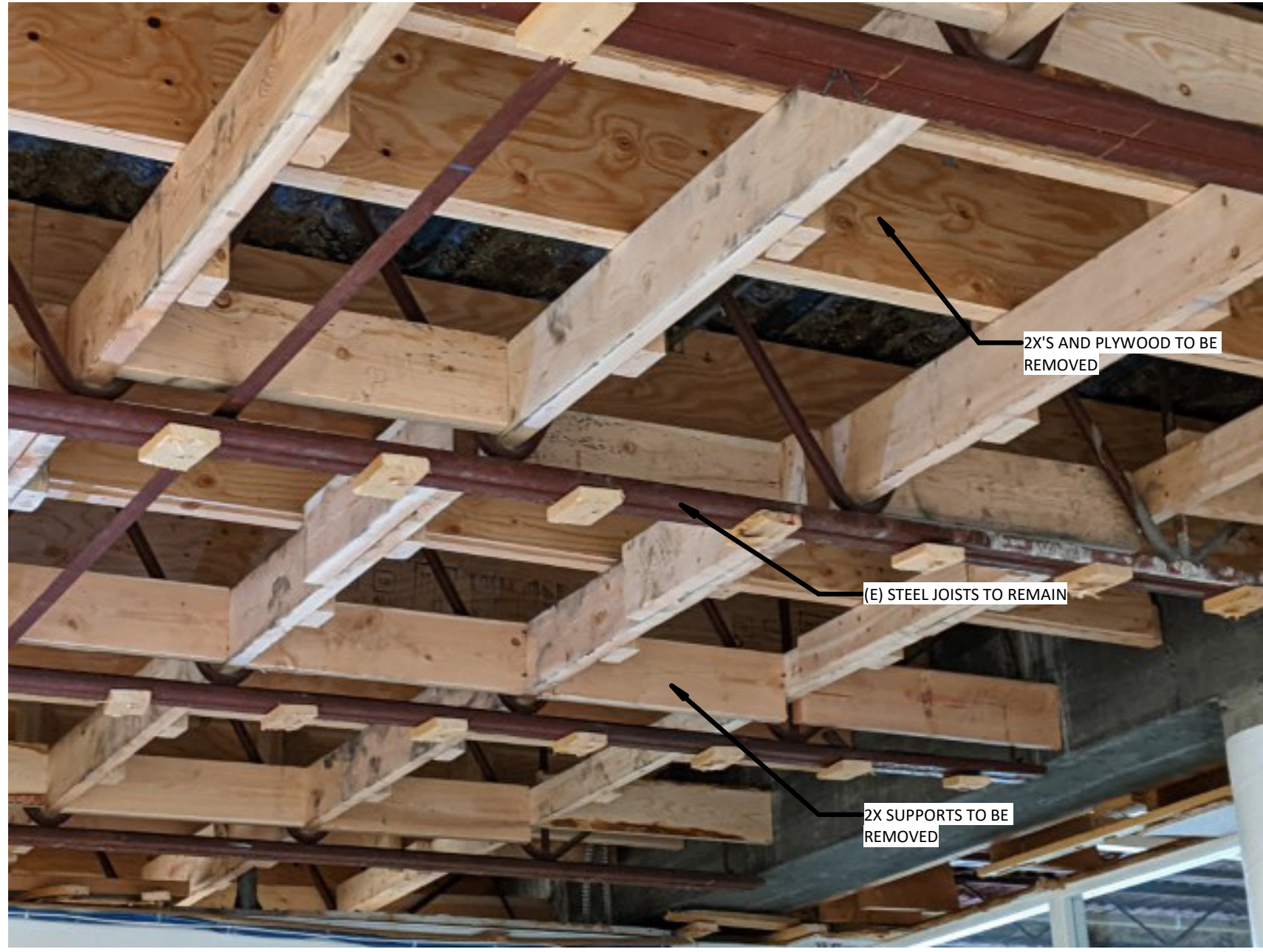
IMAGE 2 WOOD 2X AND PLYWOOD SHORING IN CLASSROOMS
