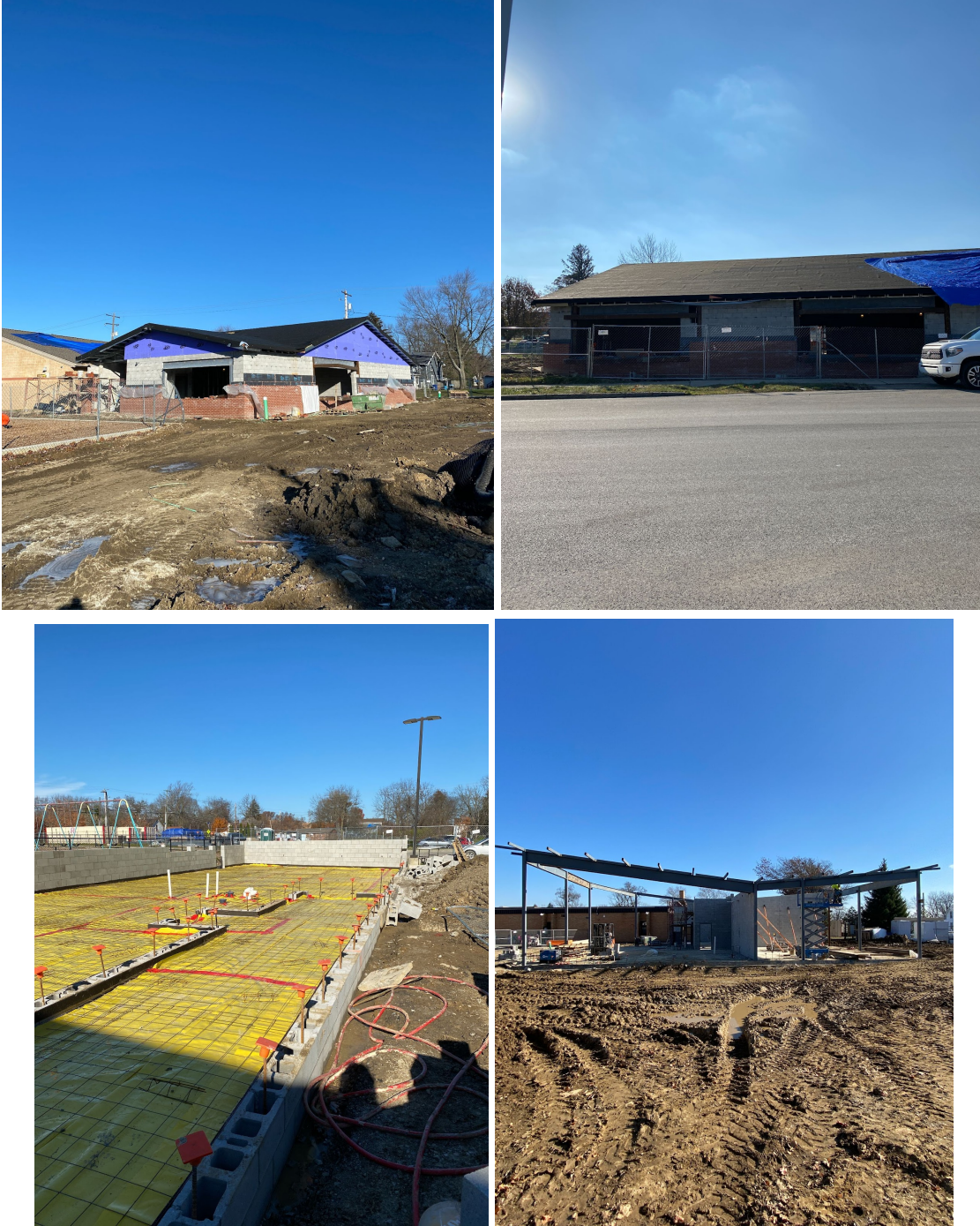
Photos of construction at Conger (top) and Woodward (bottom).
