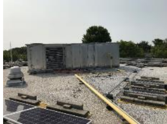
Built up stone ballast roof
