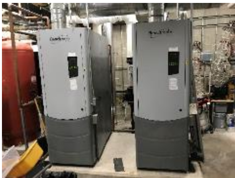
Condensing Boilers
