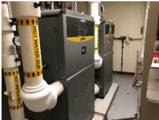
Condensing Boilers
