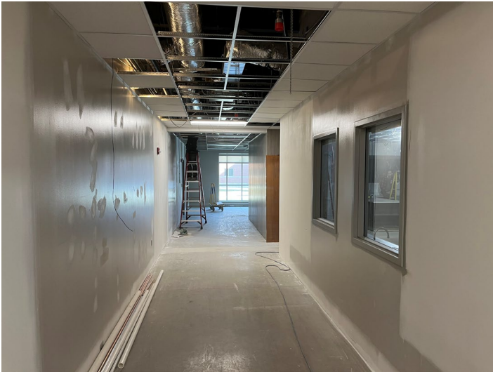
Drywall/Overhead work in Learning Center
