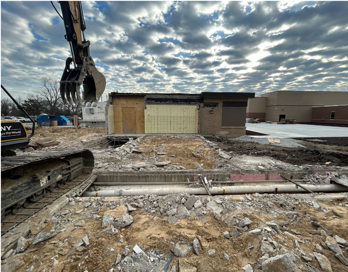
Demo of Main Entrance/Admin Area
