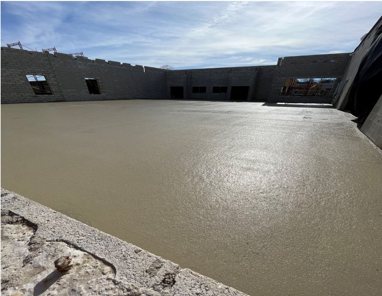
Concrete Slab in Cafeteria Kitchen Addition
