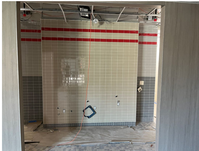
New Wall Tile in Student Restrooms
