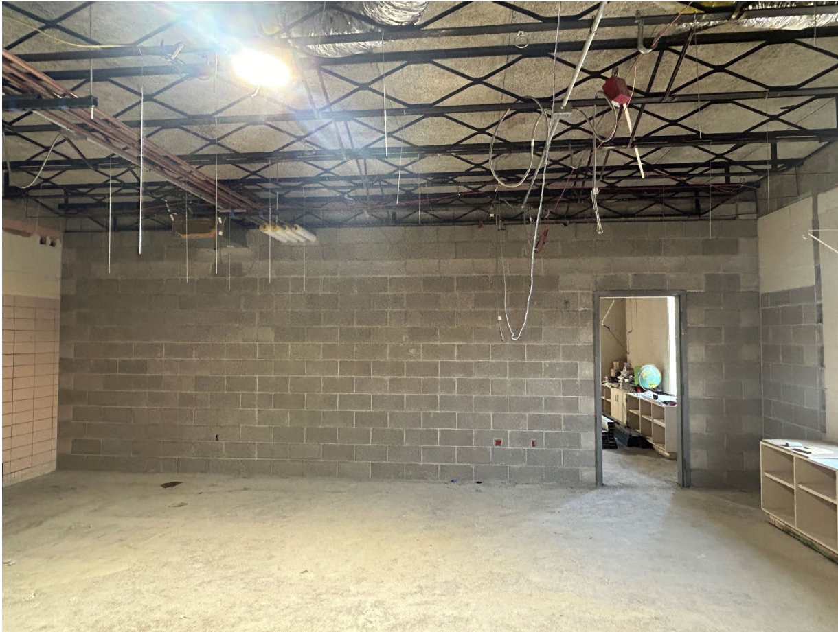
Interior CMU Installation for 3 rd and 4 th Grade Classrooms
