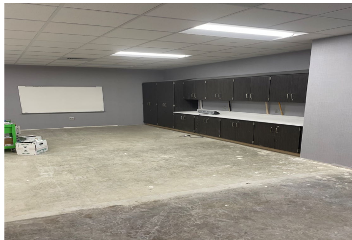
New Casework Installation
