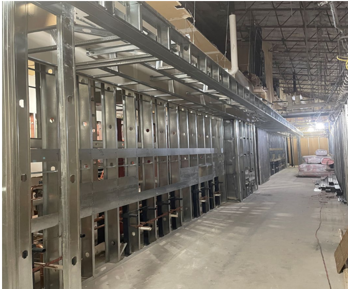
Metal Stud Framing for New Bathrooms
