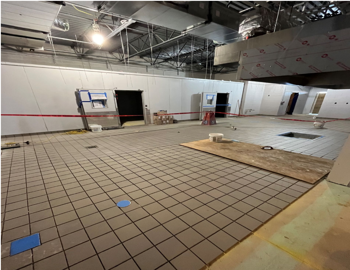
Quarry Tile Installation
