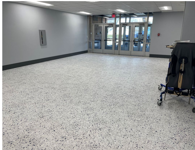
LVT Flooring in Unit C Lobby
