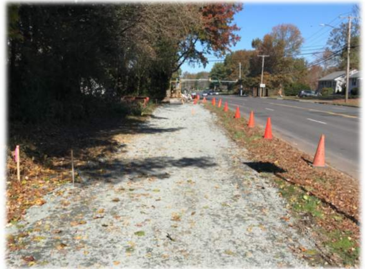
Trout Brook Trail - Phase 7 Under Construction
